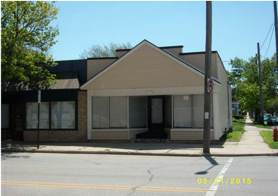
Properties in surrounding blocks; vacant or underutilized.
