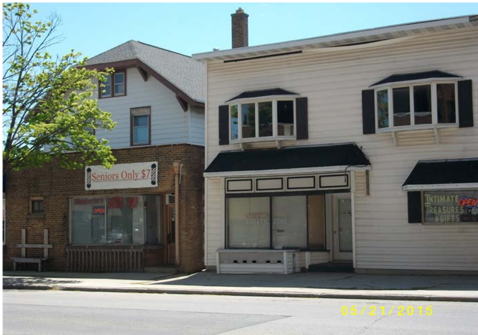
Properties in surrounding blocks; deteriorated conditions.
