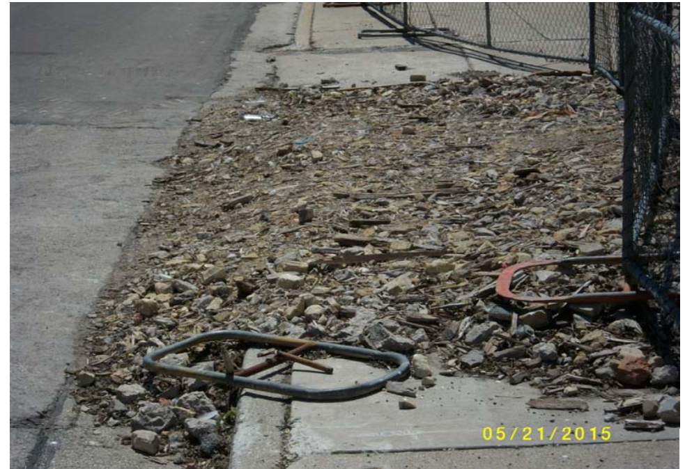
Crushed brick, wood, and other materials left as driveway approach.
