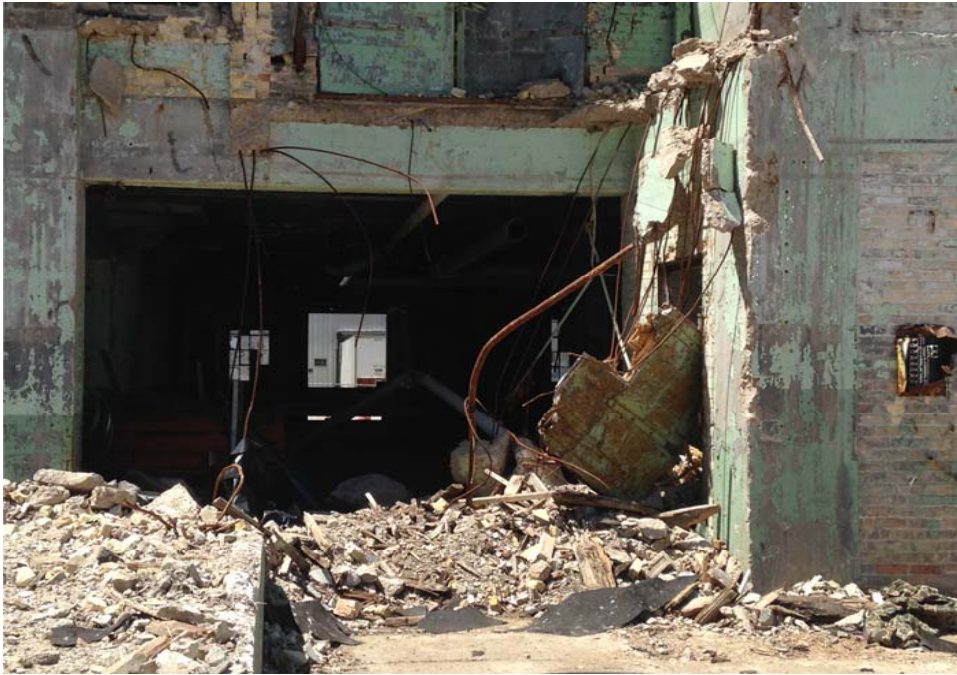
Exposed, partially demolished walls.
