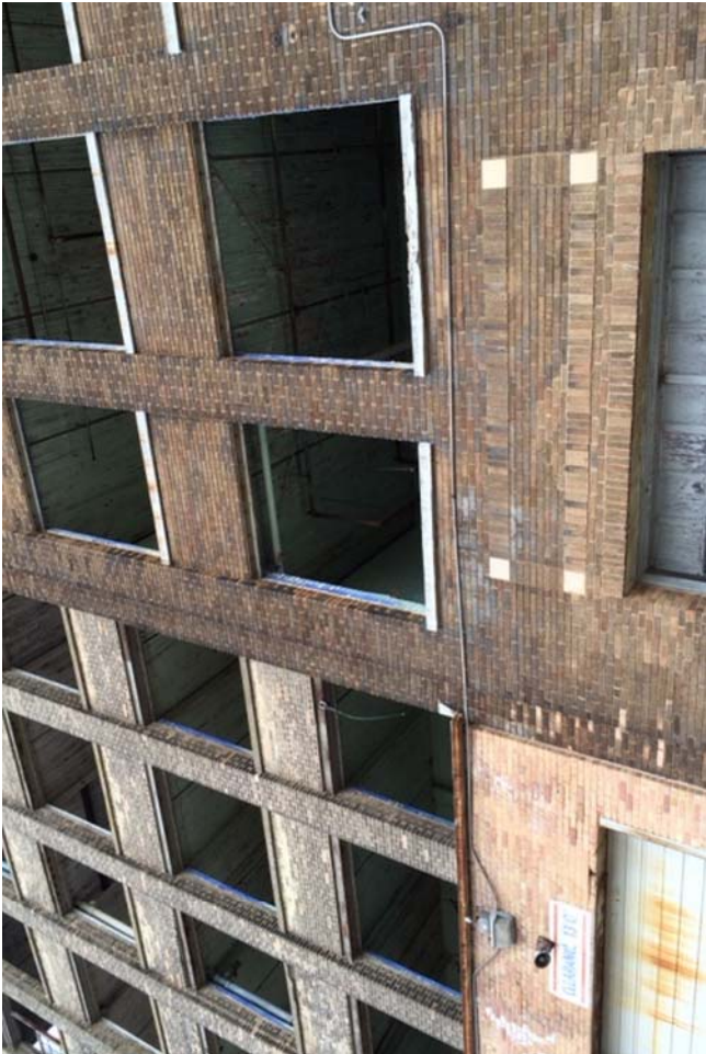
#11 - Partial demolition of building on southern portion of property
