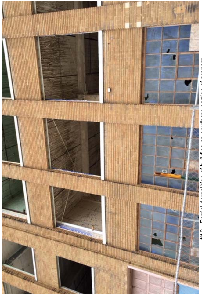
#10 - Partial demolition of building on southern portion of property
