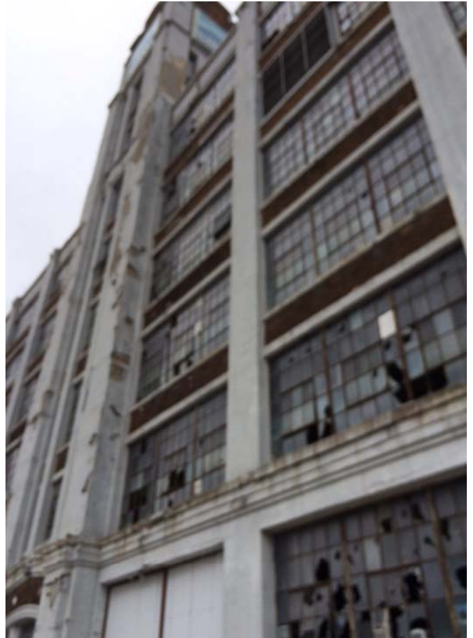
#4 - Partial demolition of building on NE corner of property
