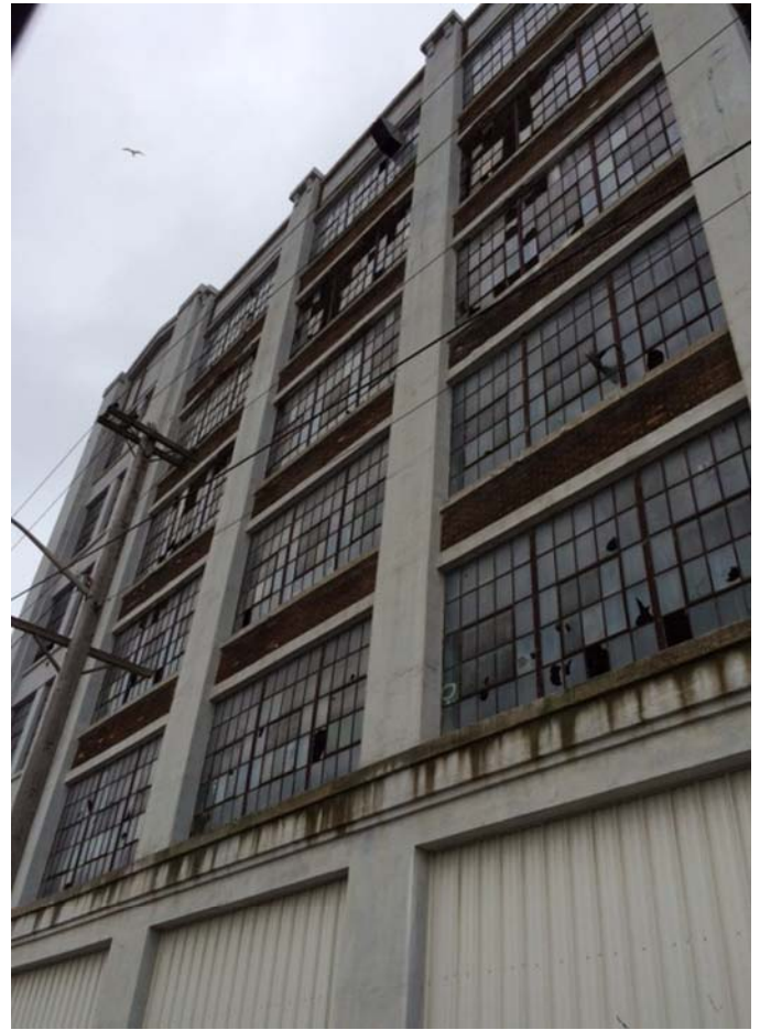
#6 - Partial demolition of building on NE corner of property
