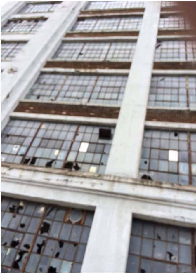
#5 - Partial demolition of building on NE corner of property
