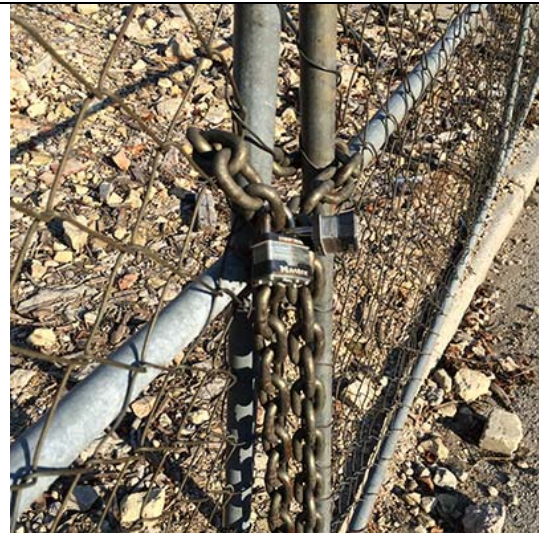
Padlock securing gated entrance to Site.
