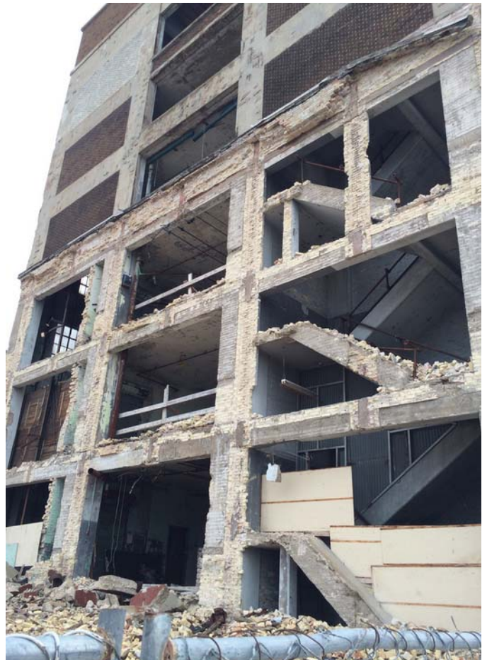
#11 - View of building exterior on north side of property
