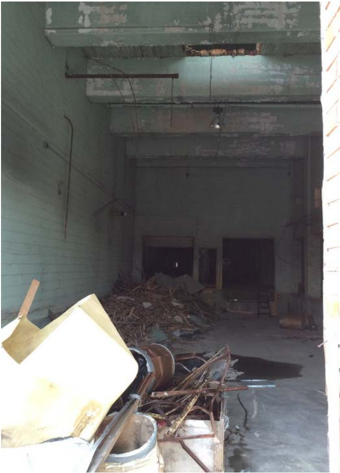
#21 - View of S loading dock, looking east from 16th St
