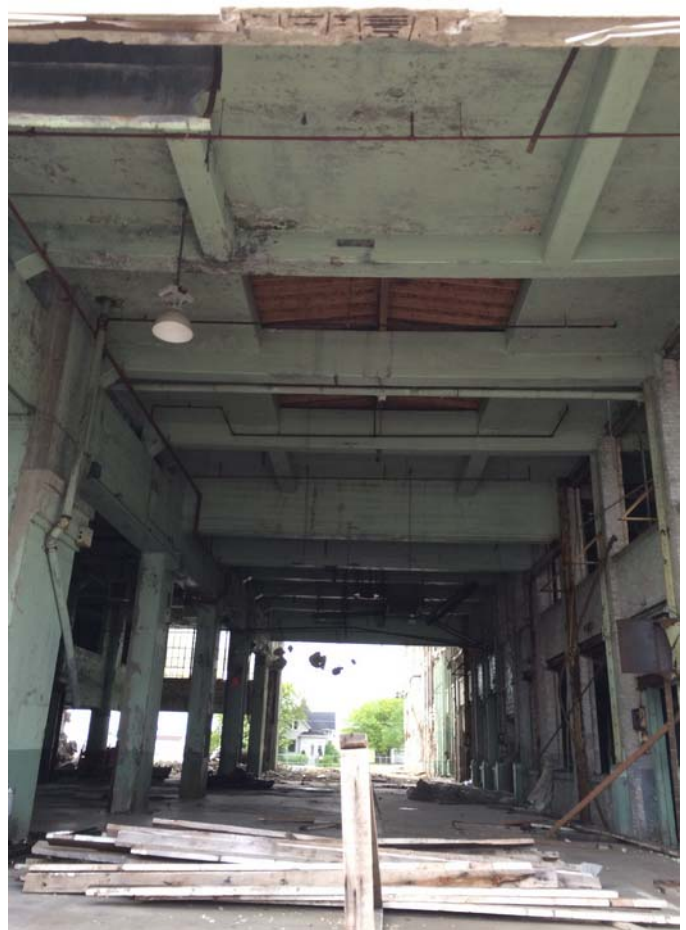
#18 - View of bldg interior, looking east from 16th St
