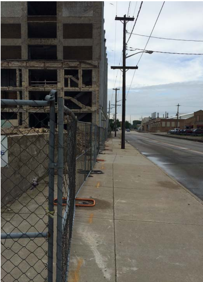
#3 - View of sidewalk on N. side of Site
