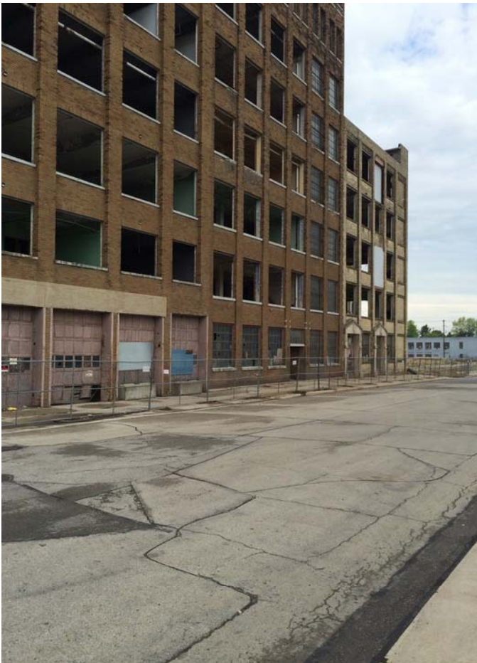
#27- View of south building, looking west from 15th St
