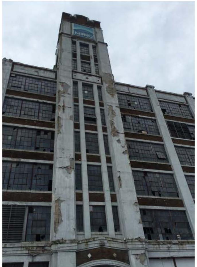
#16 - View of northwest building exterior
