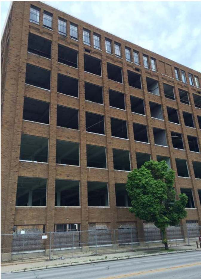
#23 - View of south side of building
