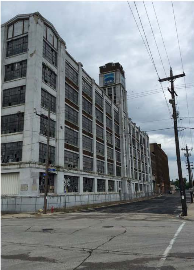
#15 - View of NE Building looking S along 16th
