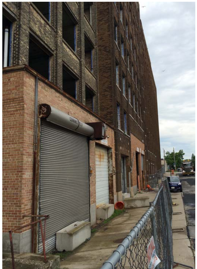
#20 - View of west side of south building, looking S along 16th St
