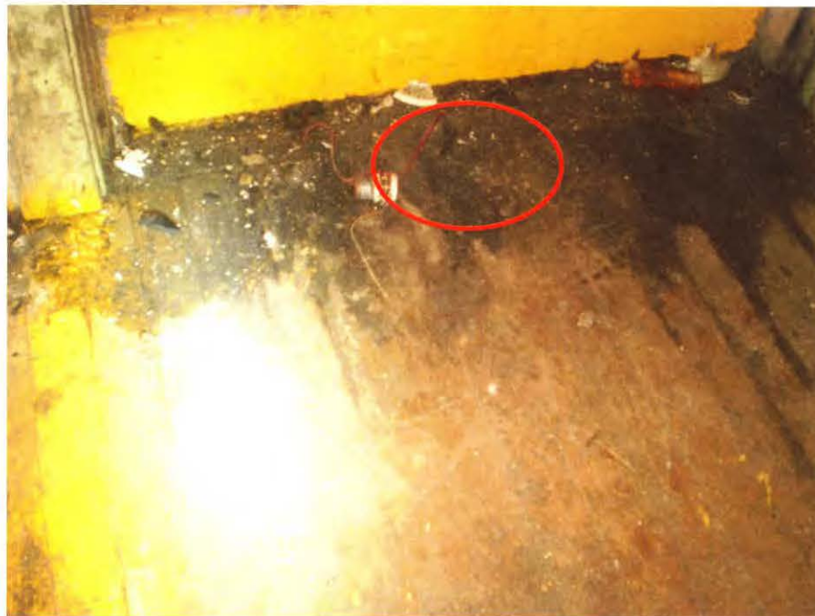
Photograph No.: 12 Photographer: Caitlin Ruza Area: Bldg I-Transformer TDD Number: TO-05-10-12-0002 Contract: EP-S5-10-10, OTIE Date: January 24, 2011 Site Name & Location: Mirro-Spirtas Site, Manitowoc, Manitowoc County, Wisconsin Photograph Subject: MS-WP-7 collected from stained area outside of entranceway to the transformer room in Building I (approximate sample area shown)
