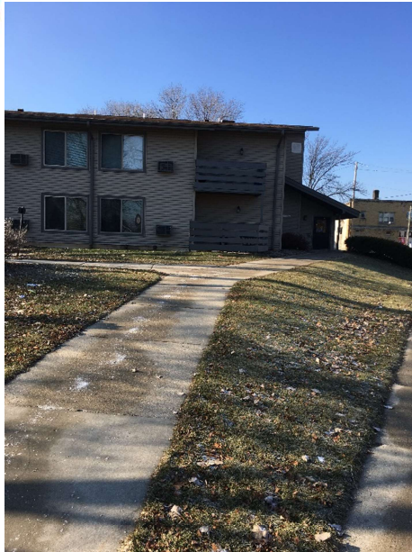
Looking to the west along W. Atkinson Ave, limited work area for remediation and apartment access updates
