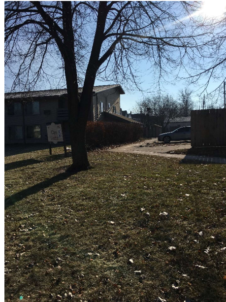
Looking to the south from W. Atkinson Ave, limited work area for remediation
