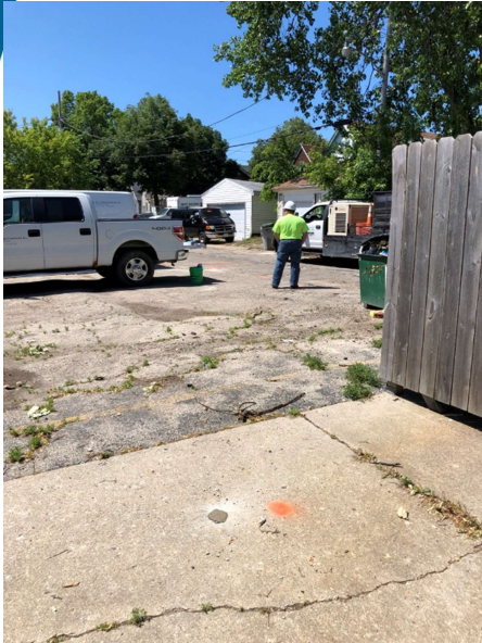
Looking to the south along alley, limited remedial work area
