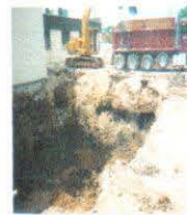
CONTAMINATED SOIL EXCAVATIONS
