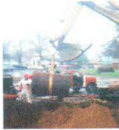
UST / AST Removal
