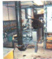
REMEDIATION SYSTEM CONSTRUCTION
