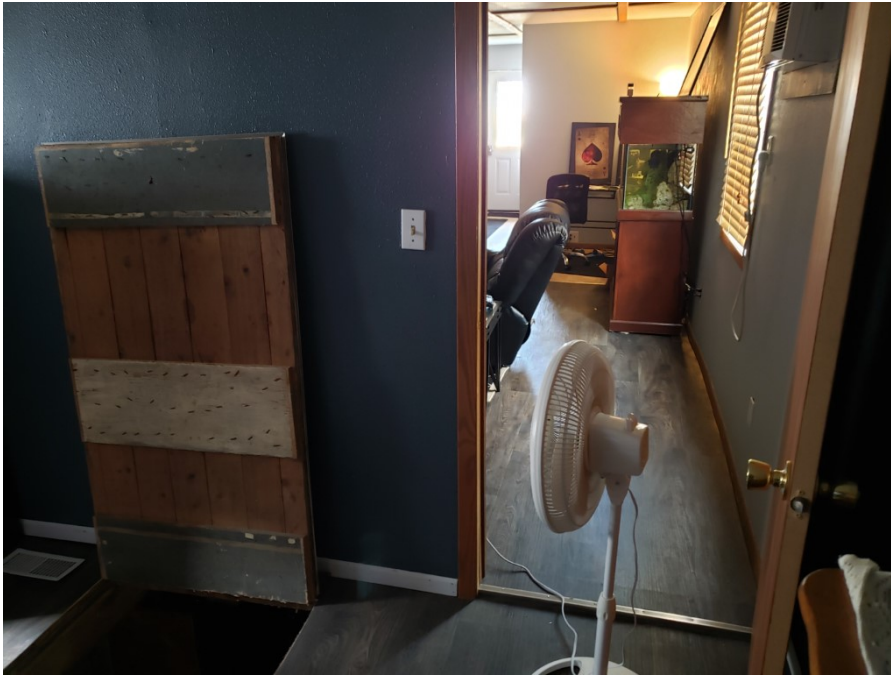
Photo 3: Basement access hatch in floor of back bedroom at 725 Sextonville Rd. (9/17/20).
