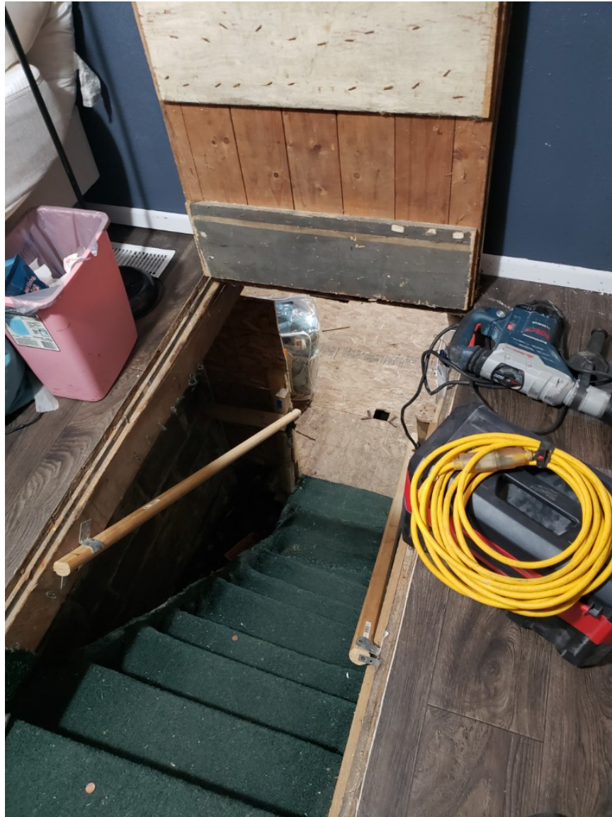
Photo 1: Basement access. August 31, 2021.
