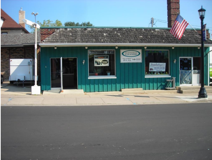
Photo 3: South end of the Platteville Cleaners property, covered with concrete.
