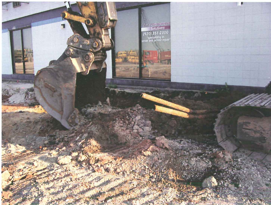
Photo 1: Initial Excavation - view looking northwest.
