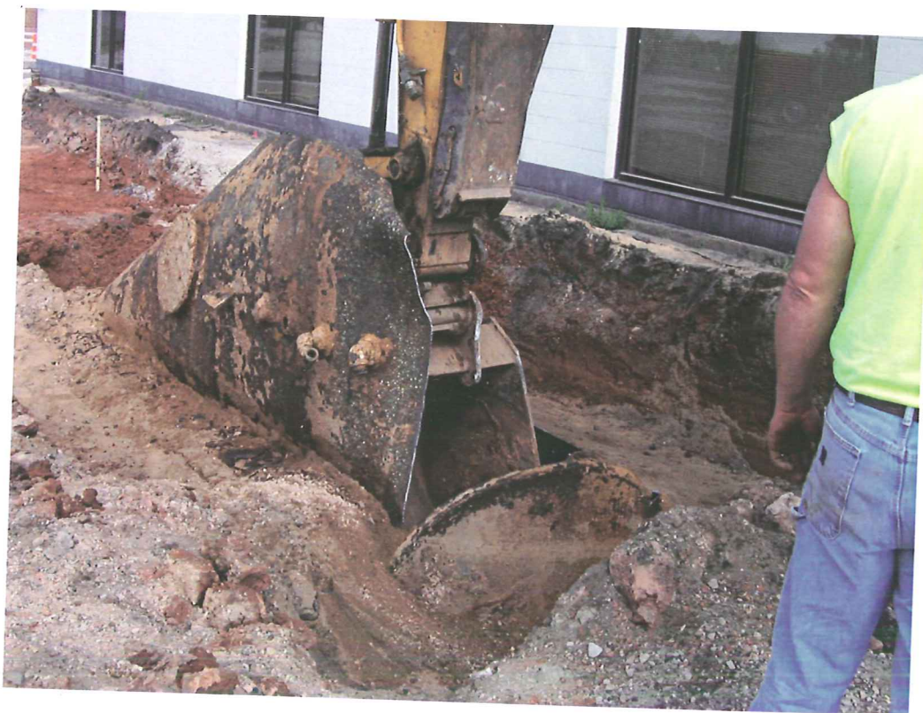
Photo 13: UST removal - view looking northwest.
