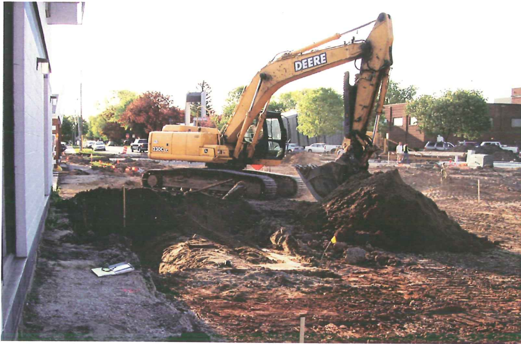
Photo 5: Top of UST exposed - view looking west.
