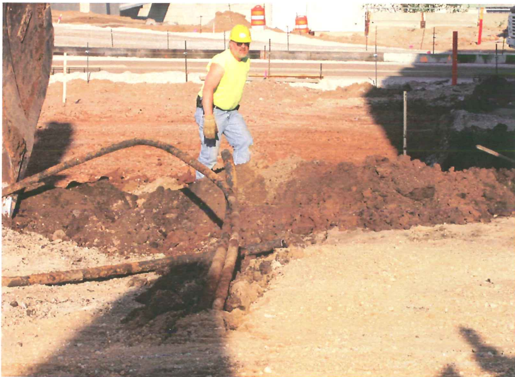
Photo 4: Piping Removal (vent pipe and fill pipe) - view looking west.
