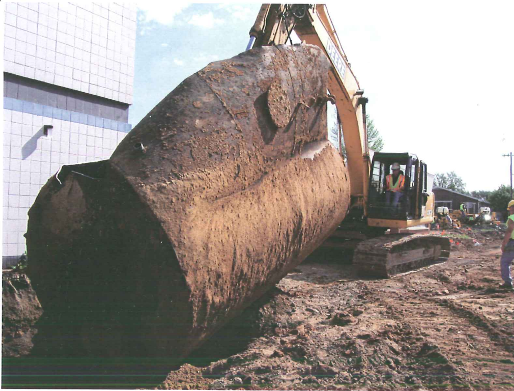
Photo 15: UST removed from ground - view looking northeast.
