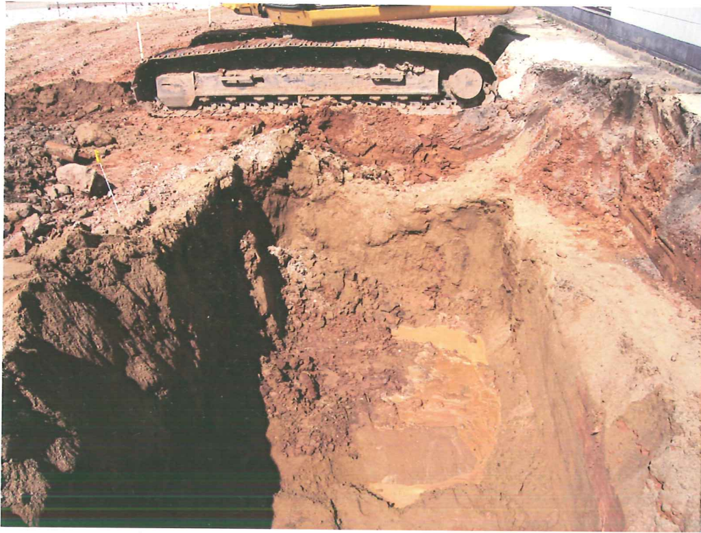
Photo 17: West end and center of excavation - view looking west.
