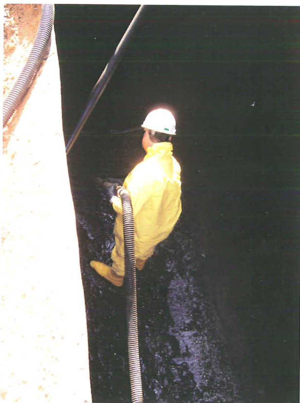
Photo 10: ESP personnel cleaning UST with vacuum truck - view looking east.
