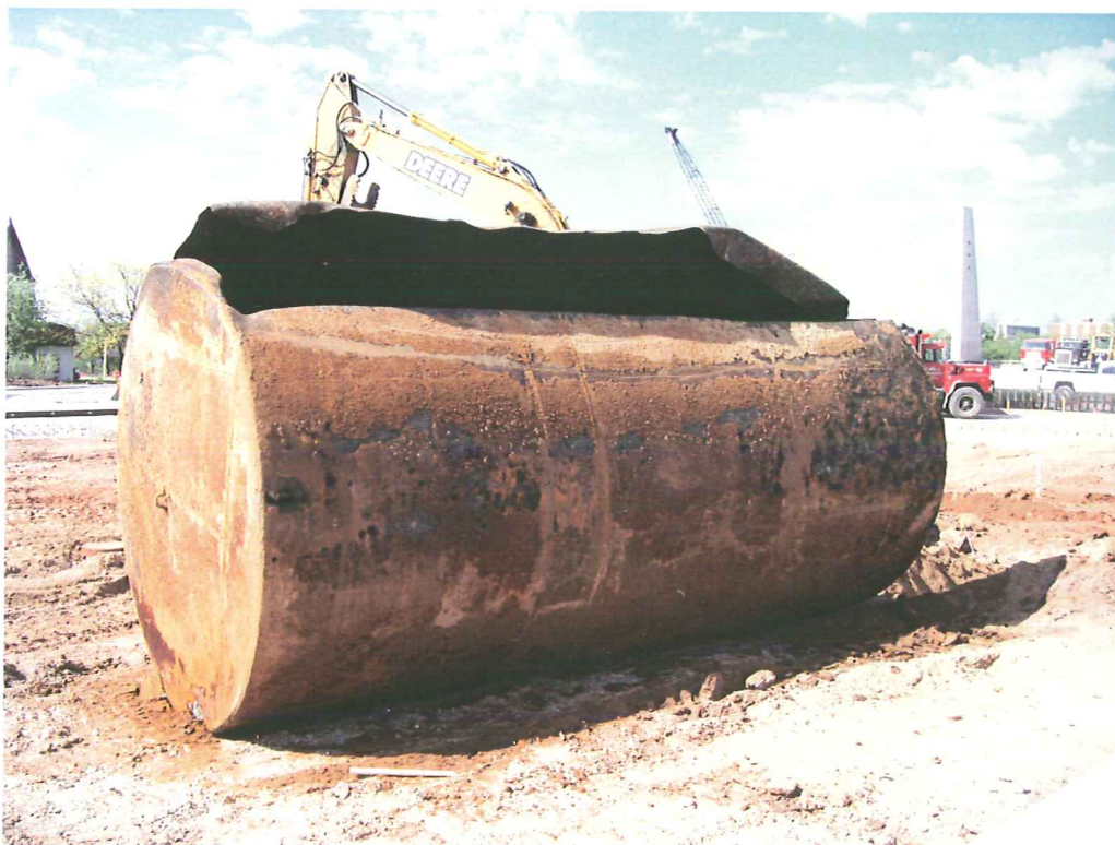
Photo 16: UST ready to load for disposal - view looking southwest.
