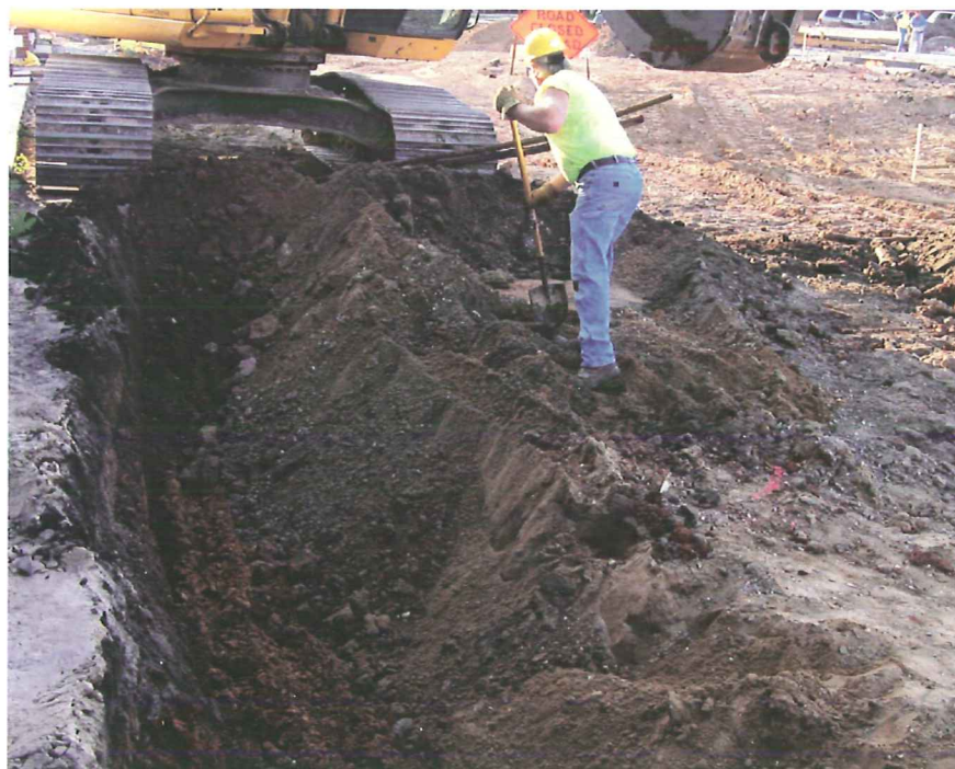
Photo 2: Exposing top of UST - view looking east.
