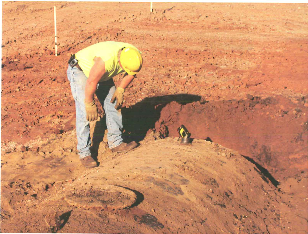
Photo 6: UST atmosphere monitoring prior to cutting – view looking west-southwest.
