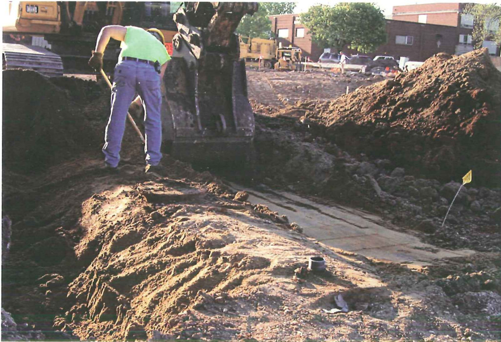
Photo 3: Final Cleaning of UST top - view looking east.
