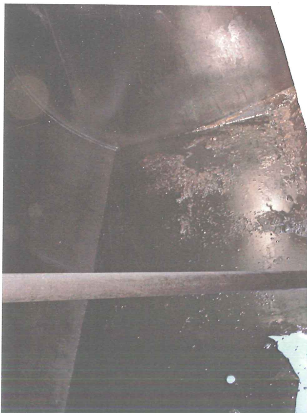
Photo 9: Interior of UST. Sludge and liquid in bottom of UST prior to vacuum cleaning - view looking west.
