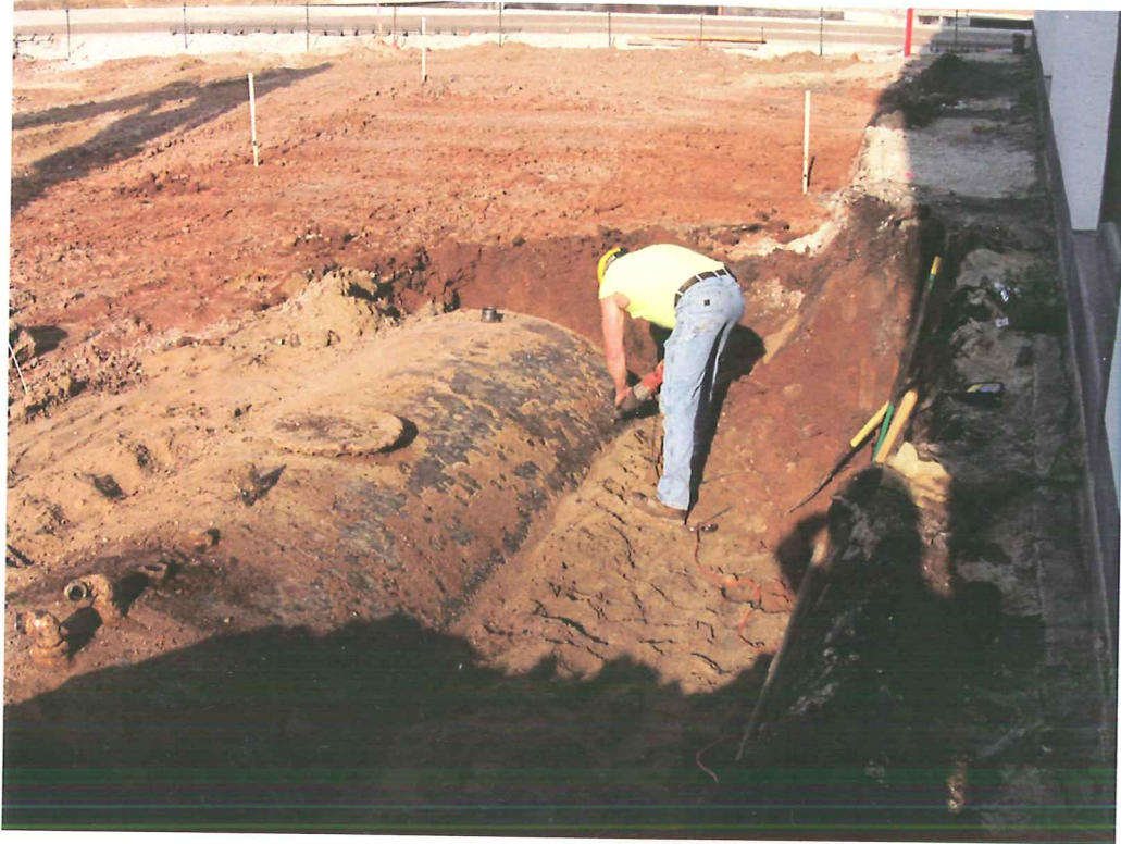
Photo 7: Cutting UST open using Sawzall - view looking west.
