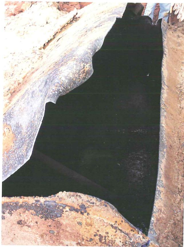
Photo 8: UST following opening by backhoe - view looking west.
