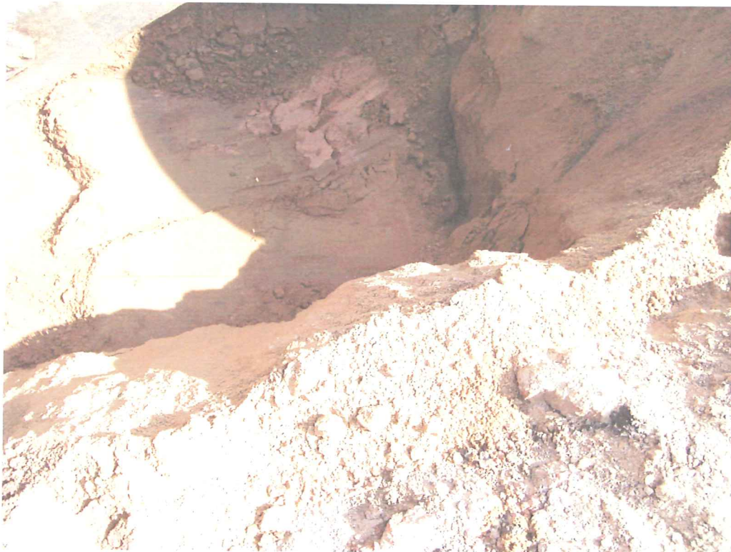
Photo 18: East end of excavation - view looking northeast.
