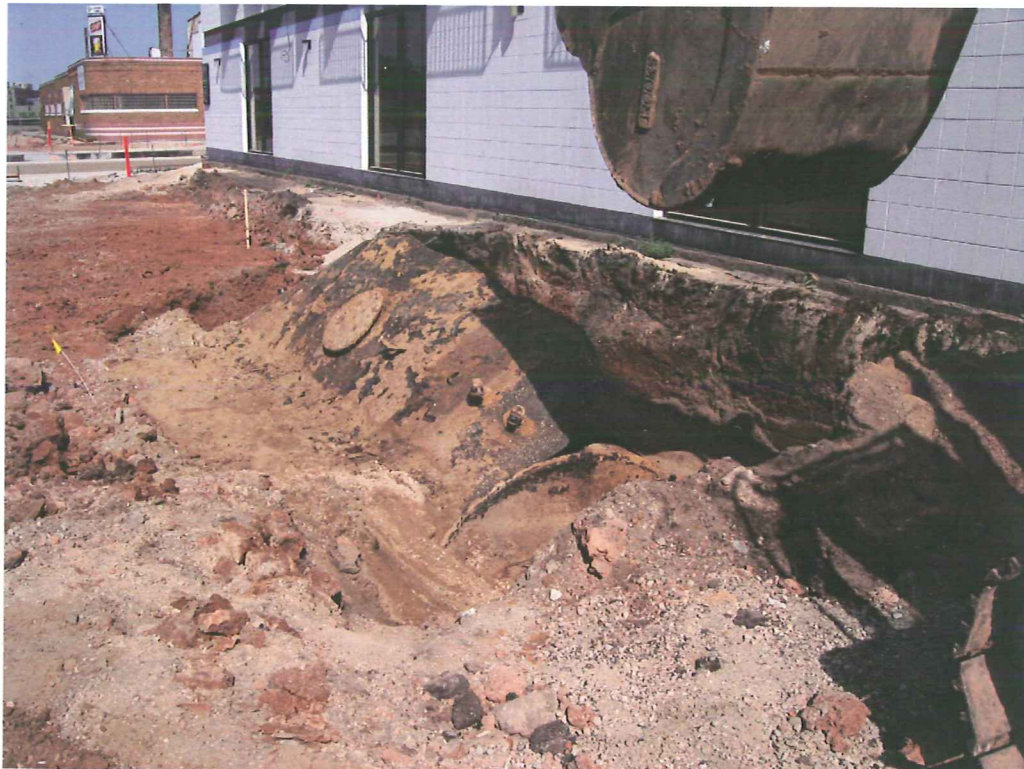
Photo 12: UST ready to remove - view looking northwest.
