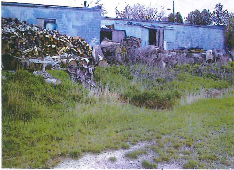
View to the southeast, west side of 8655 N. 43 rd Street. Discharge area visible in the center of the photo.
