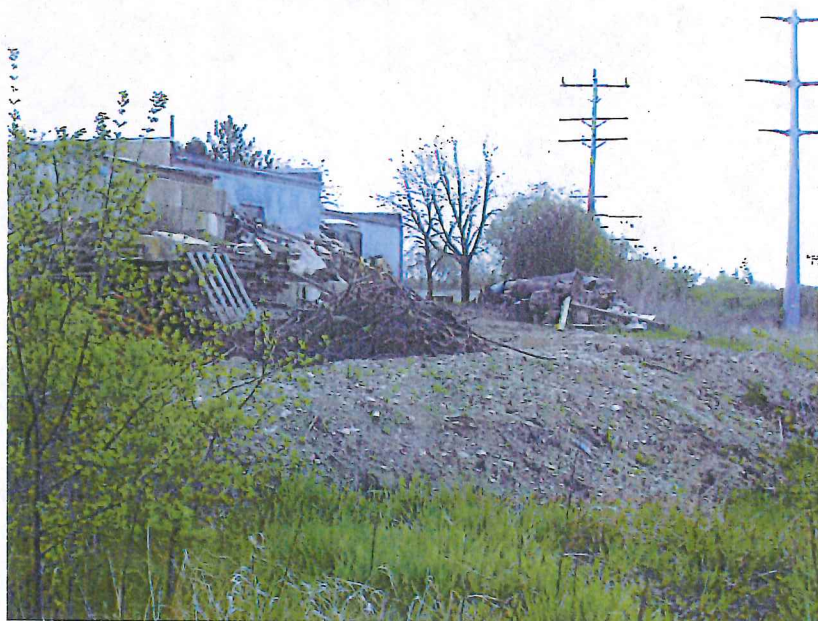
View to the south, west side of 8655 43 rd Street lot. Two building corners visible on the left.
