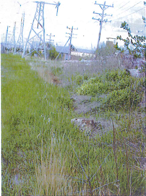
View to the north, west side of 8655 N. 43 rd Street. Discharge flows from the center of the photo towards the bottom of the photo.
