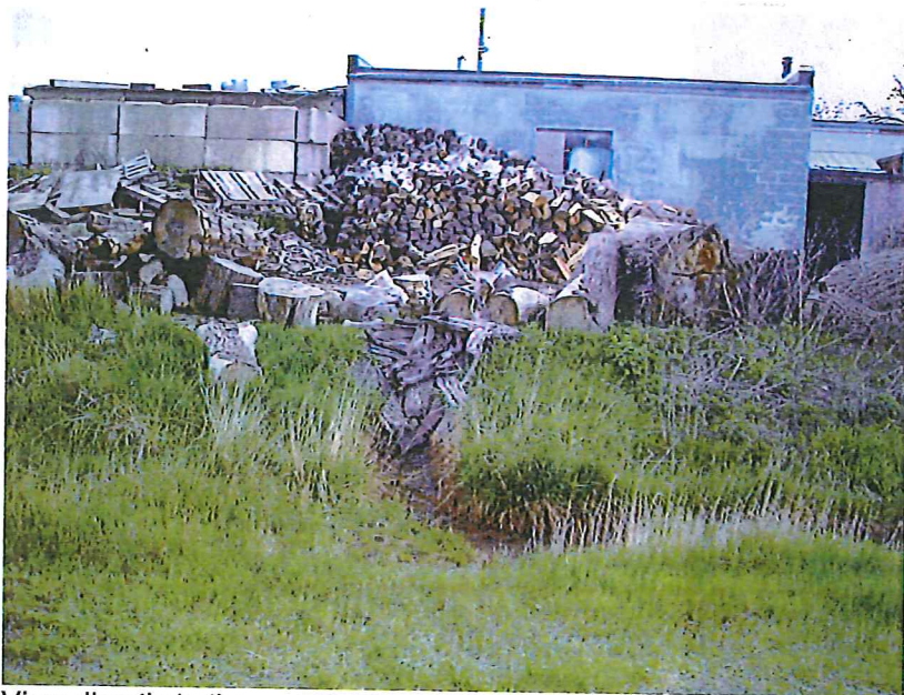
View directly to the east, looking at the west side of 8655 43 rd Street. Discharge area in the middle of the photo.
