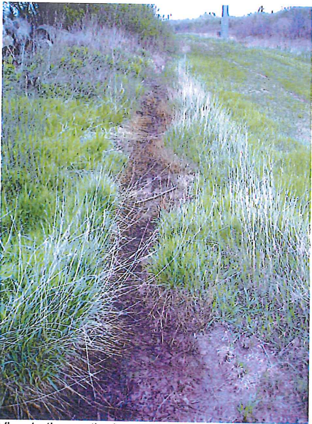
View to the south along east side of ROW.
