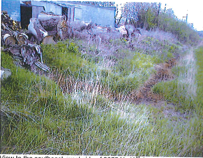
View to the southeast, west side of 8655 N. 43 rd Street. Shows flow of discharge from under the bark and debris to the west, and then southward along east side of ROW.
