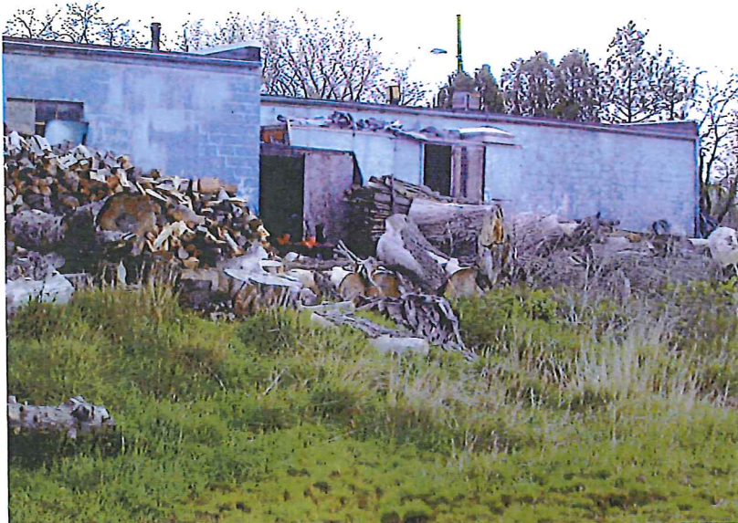
View to the southeast, west side of 8655 N. 43 rd Street.
