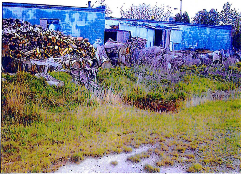
View to the southeast, west side of 8655 N. 43 rd Street. Discharge area visible in the center of the photo.
