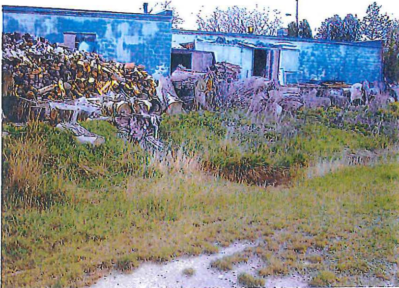
View to the southeast, west side of 8655 N. 43 rd Street. Discharge area visible in the center of the photo.
