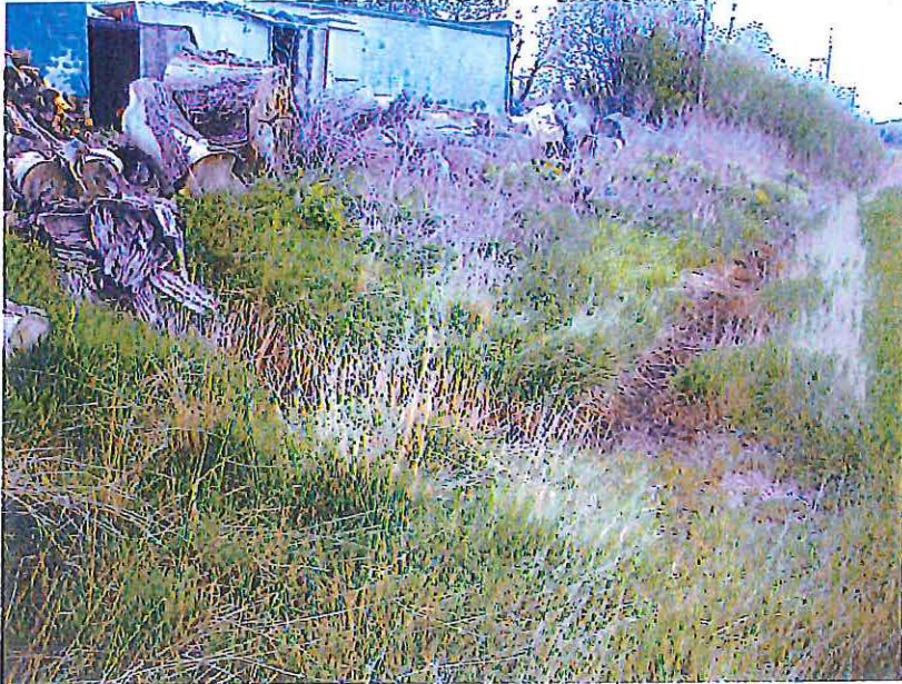
View to the southeast, west side of 8655 N. 43 rd Street. Shows flow of discharge from under the bark and debris to the west, and then southward along east side of ROW.
