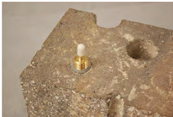
Figure 4. Installed Vapor Pin™.
