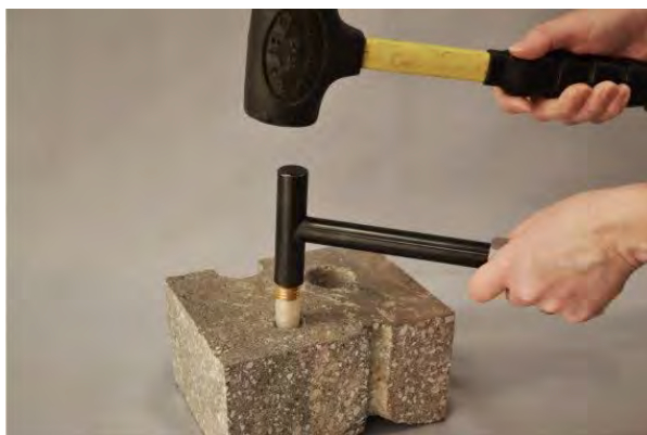
Figure 2. Installing the Vapor Pin™.
