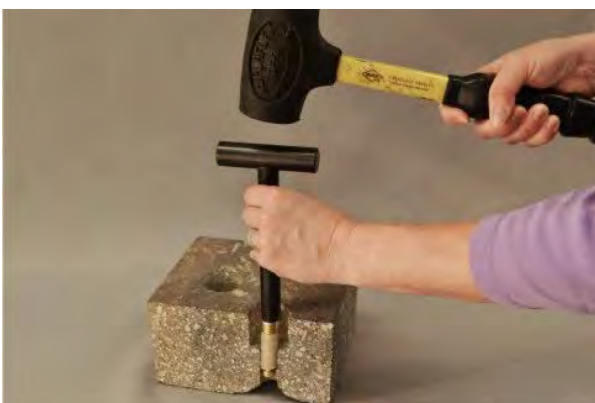
Figure 3. Flush-mount installation.
