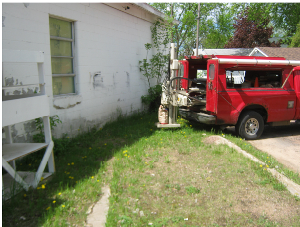
Photo #5 View looking west at location of soil boring P-13.
