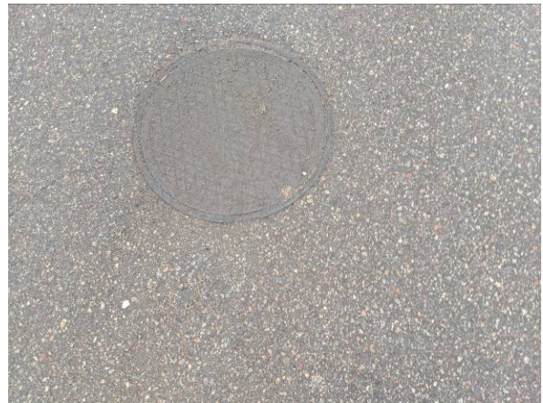
Photo #4 Photograph of manhole vapor location MH-1.
