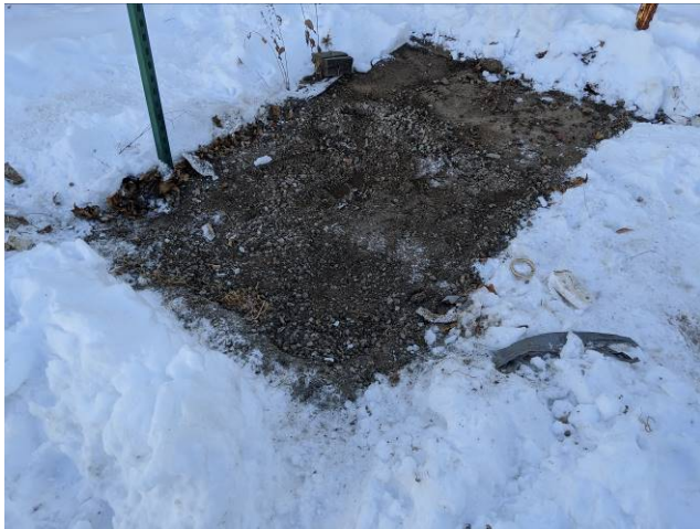
Photo #3 Photograph of temporarily capped pipping below ~ 6 inches of topsoil.
