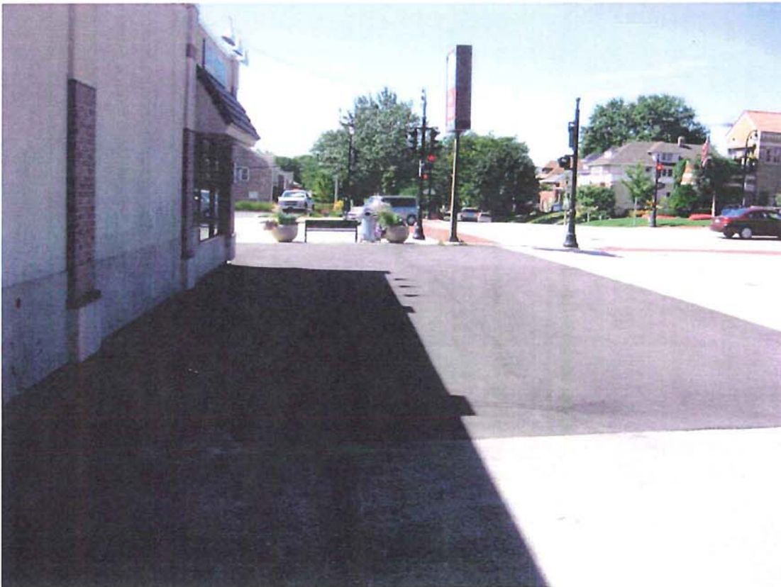
Photograph #: 2 Date: 9/8/2011 Direction: Facing West Subject: Asphalt on north side of site
