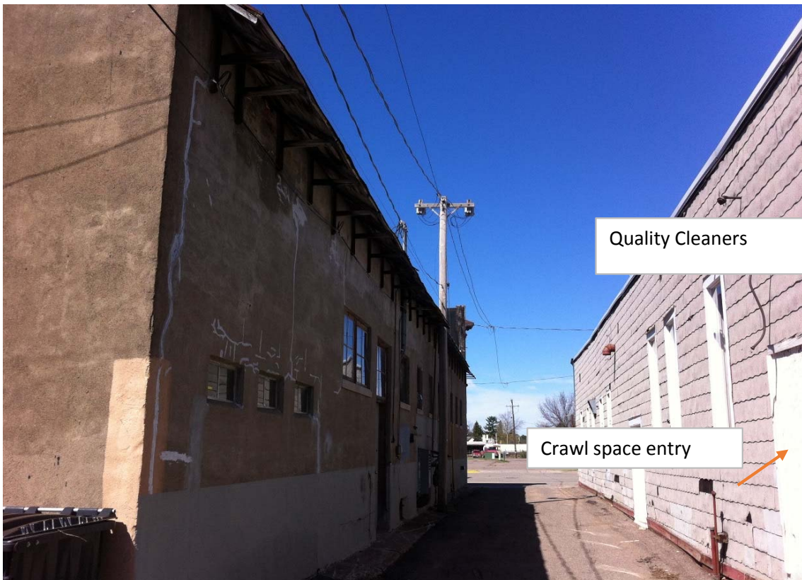
Dry cleaner building, facing west through alley
