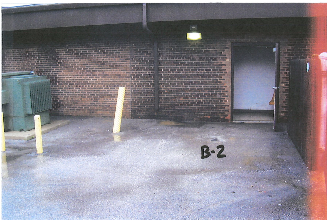
Photo Description: Pictured is the location of boring B-2, located just south of the Ruthanne's tenant space. Photo Direction: North.
