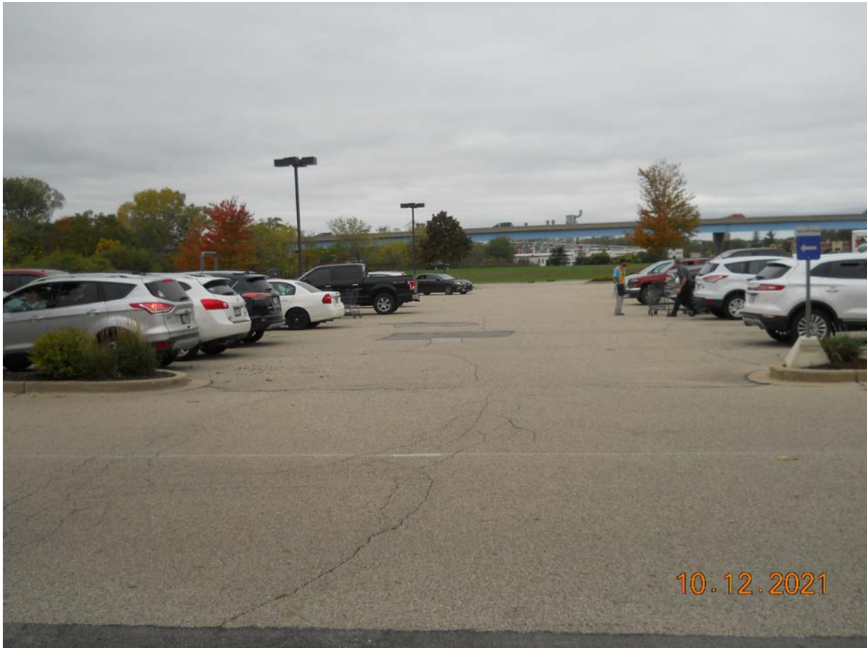
Overview of southern part of asphalt cap, facing west
