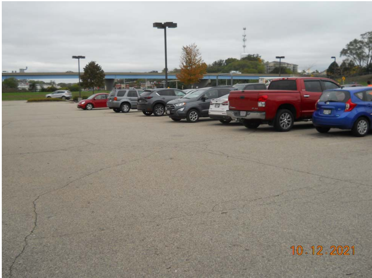
Overview of northern part of asphalt cap, facing west
