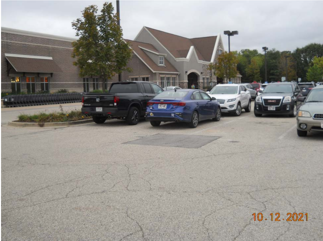
East side of asphalt cap area, facing southeast
