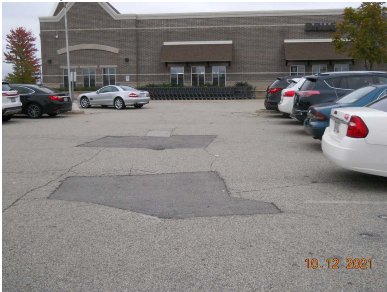
Asphalt patches installed after abandonment of remediation system
