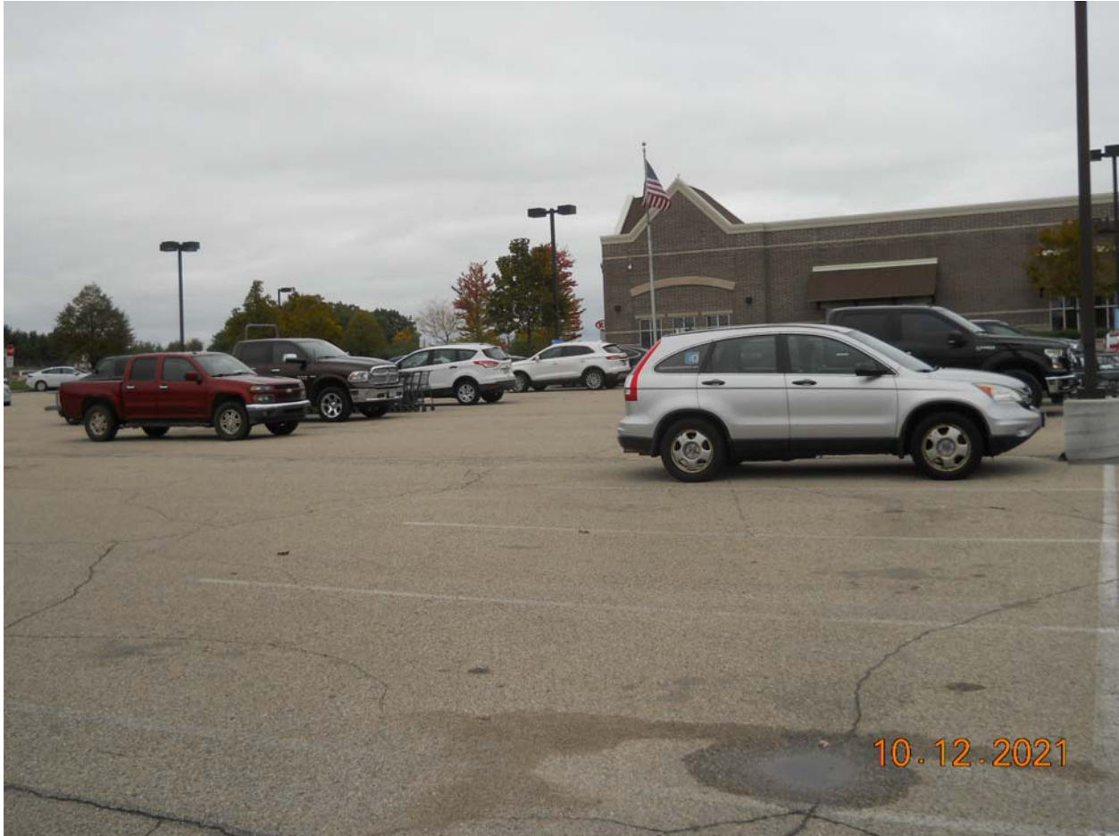
West side of asphalt cap area, facing northeast
