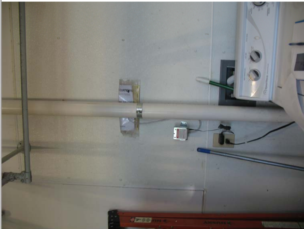
Title: Vent inside building.
