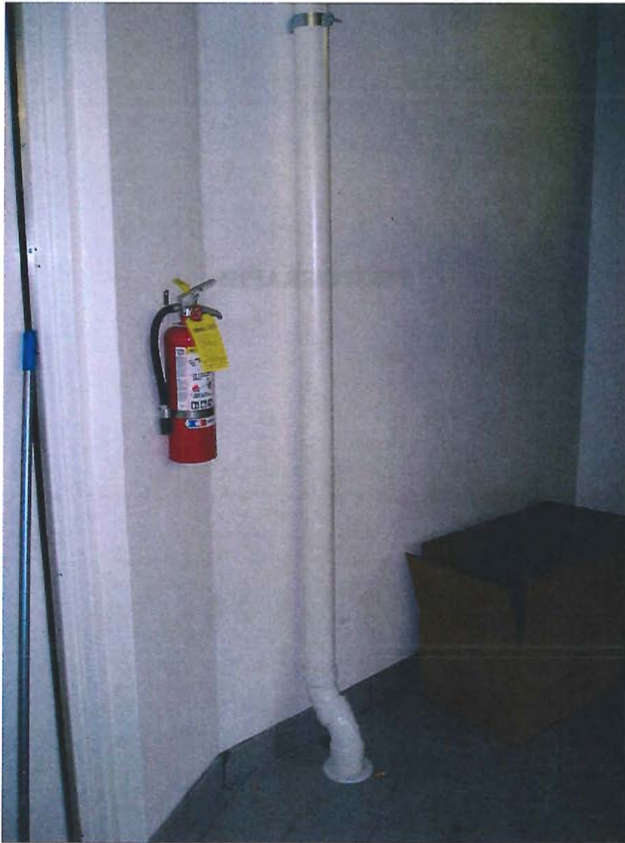
Photograph 1: Extraction Point 2. May 13, 2013
