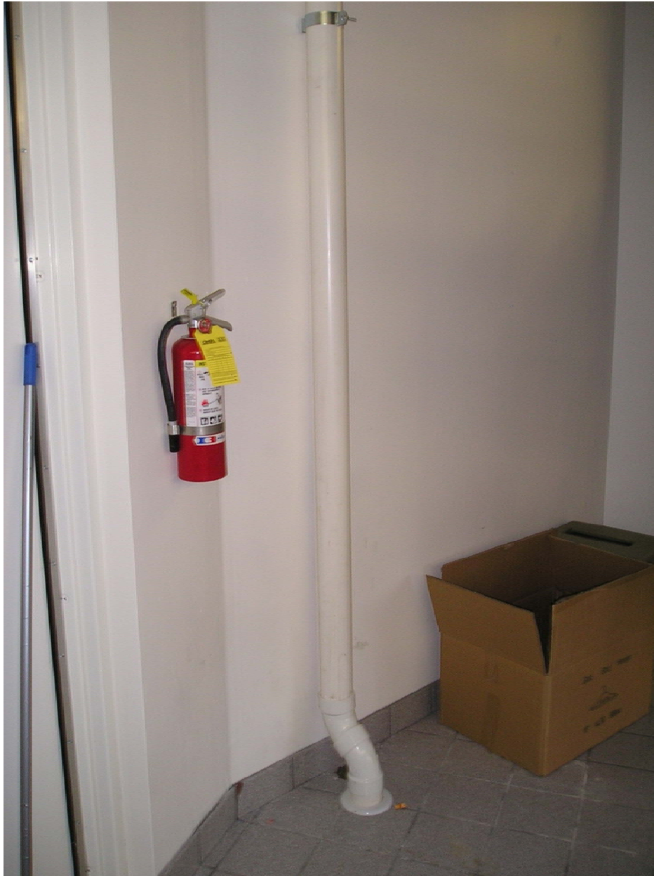
Photograph 1: Extraction Point 2. May 13, 2013
