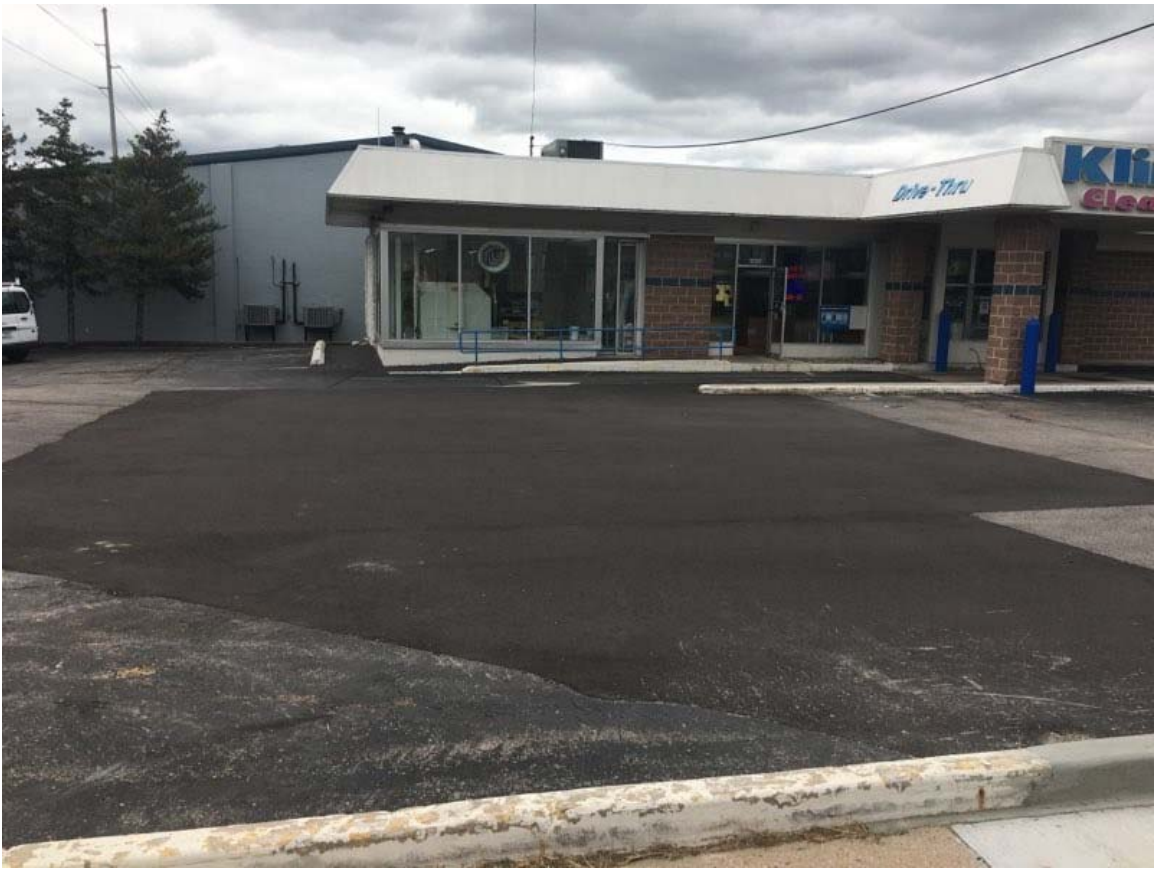
Overview of completed asphalt replacement, facing east.
