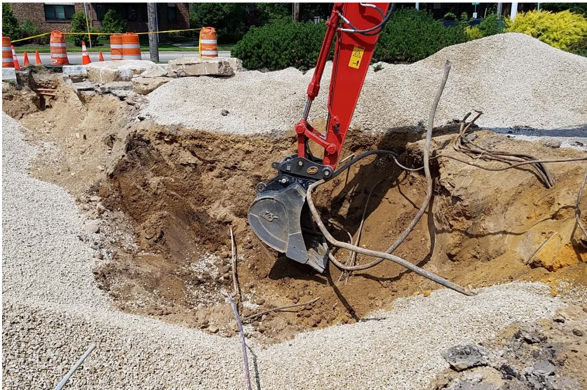
Excavator removing piping associated with former gas station infrastructure.
