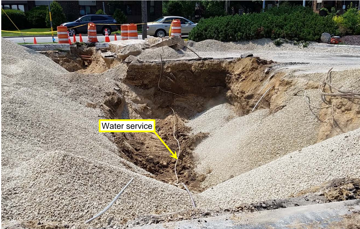
Orientation of existing water service, facing west.
