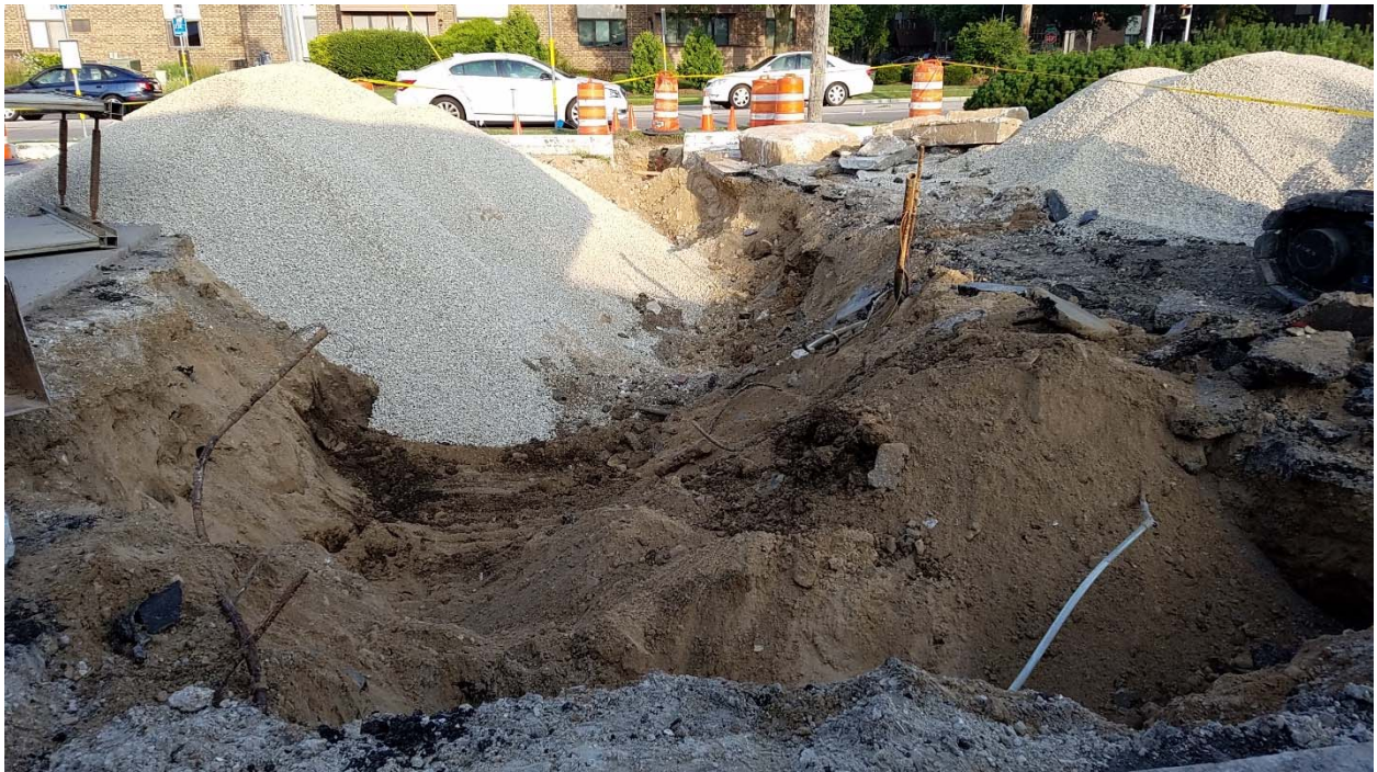
Excavation in progress, facing west.
