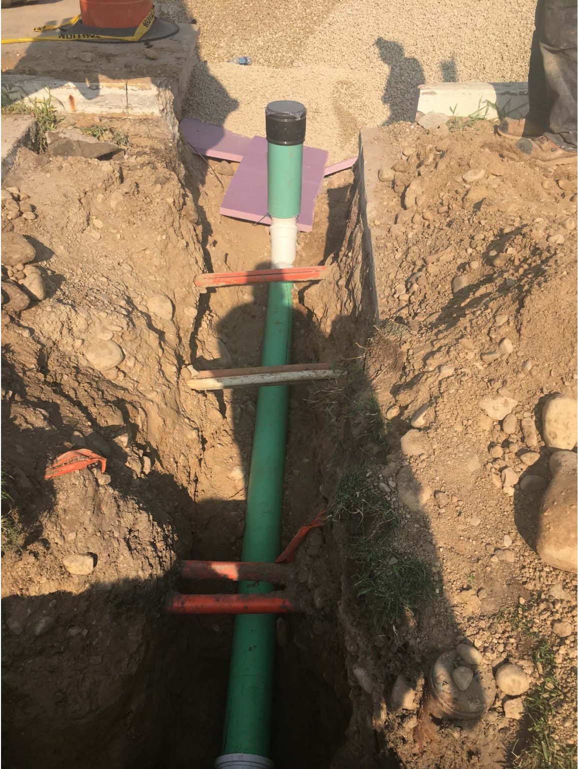
Replacement sewer lateral beneath sidewalk and terrace.
