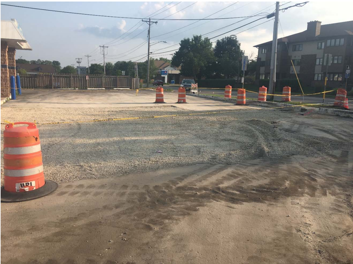
Backfilling completed, facing south.
