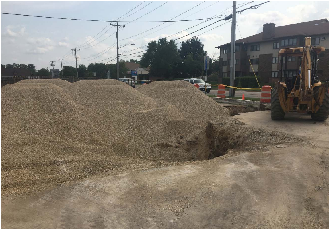
Backfilling in progress, facing south.
