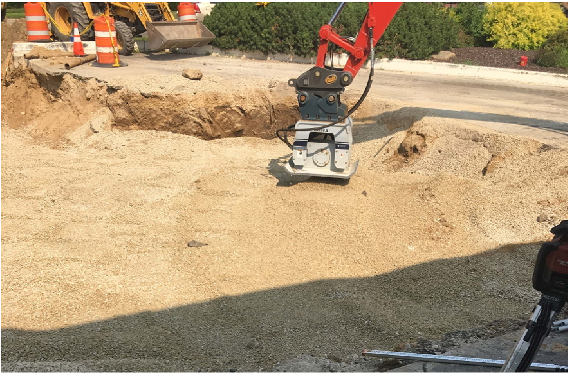
Compaction of gravel backfill.
