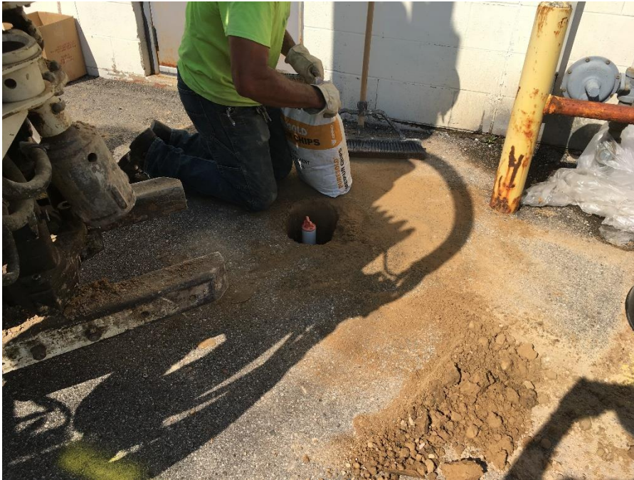
Photo 2: SVE well construction. August 5, 2019.
