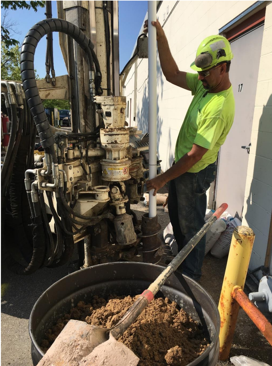
Photo 1: Installation of SVE wells. August 5, 2019.
