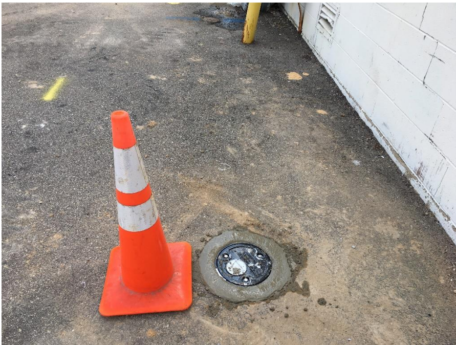
Photo 3: Completed SVE well. August 5, 2019.
