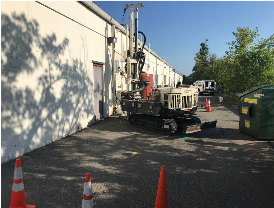
Photo 1: Installing SVE well SVE-3. Date: 8/5/19 Photo Direction: North
