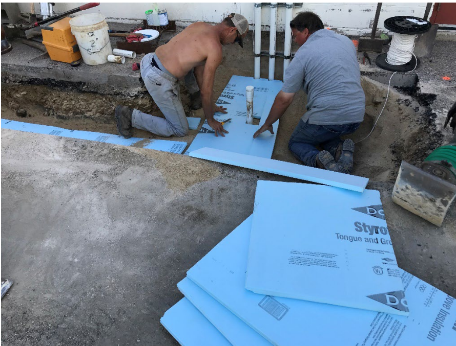
Photo 4: Installing insulation over SVE piping. Date: 7/28/22 Photo Direction: West
