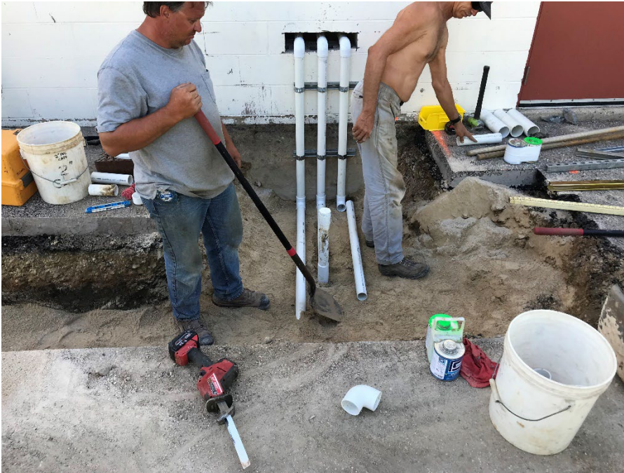
Photo 3: Installing 2-inch diameter PVC SVE piping. Date: 7/28/22 Photo Direction: West
