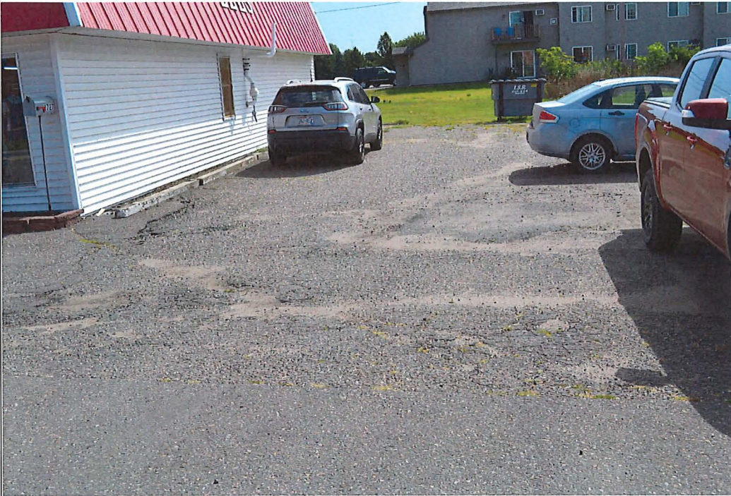
Title: Side of the building showing the cap. This photo is facing northeast.
