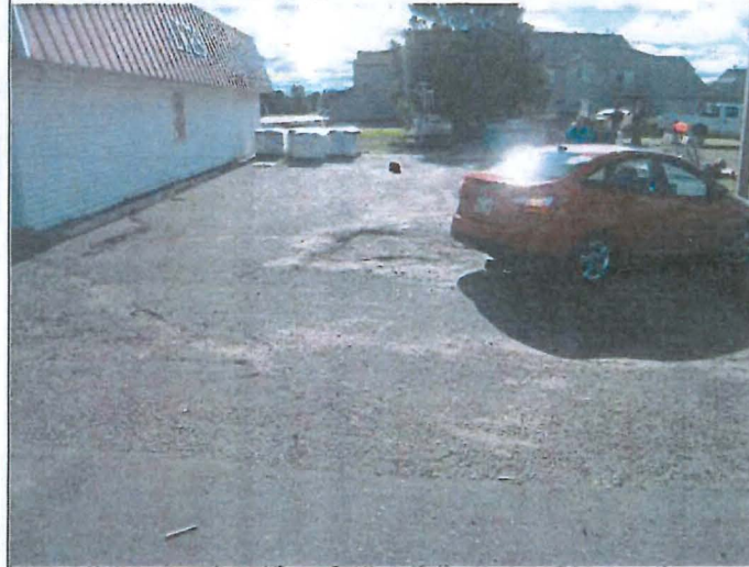
Title: Asphalt Cap 2 / Concrete Cap 3 South of Building
