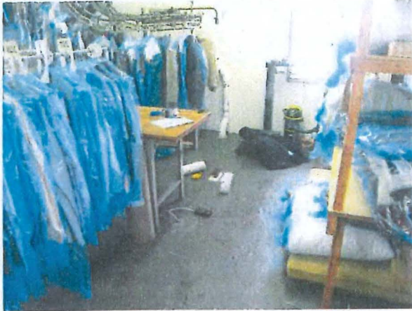
South vapor mitigation system inside Lee's Cleaners building, one floor penetration.
