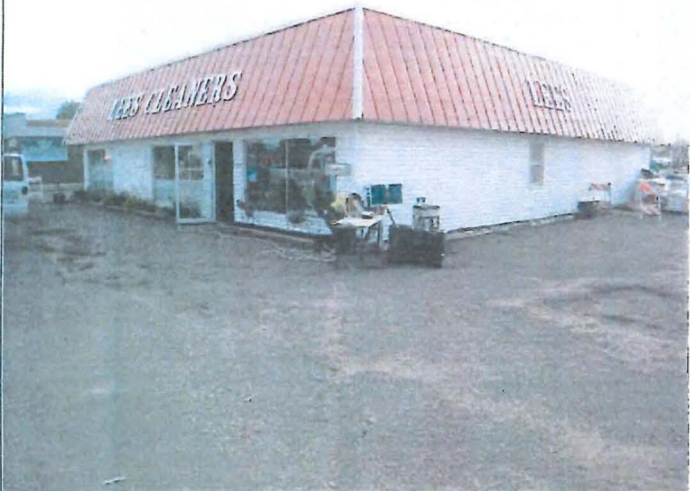
Title: Concrete Cap 1 (Building) & Asphalt Cap S & W of Building
