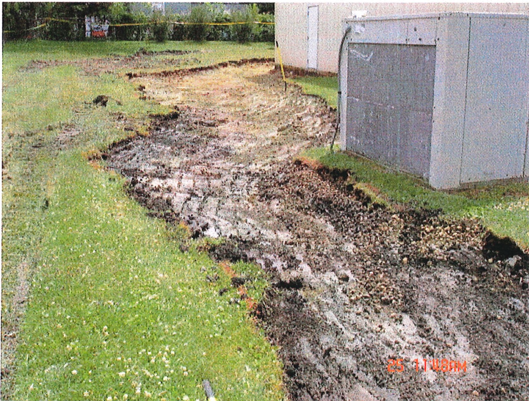
Excavation coming around northeast corner of building
