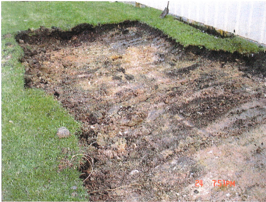
Impacted soil was excavated
