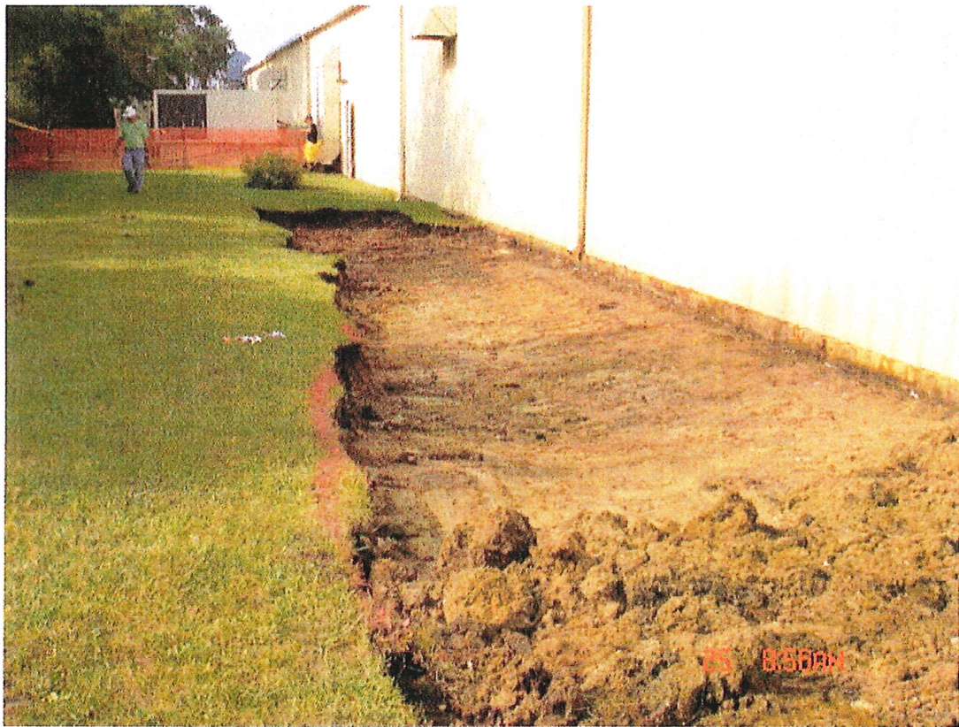
Area excavated on east side of building
