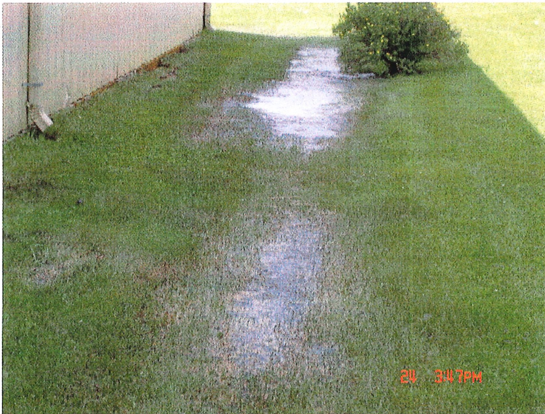
Looking north on east side of building
