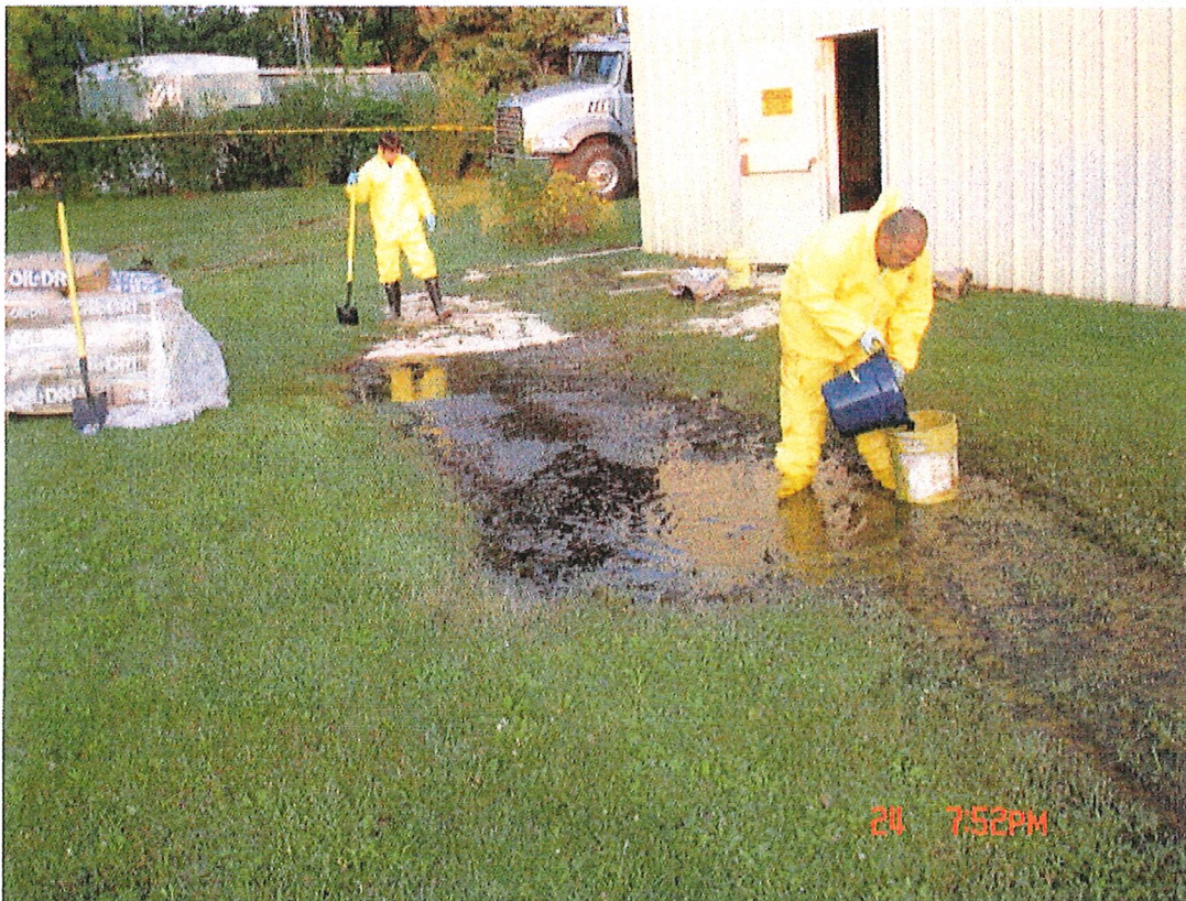
Large pool of liquid being recovered using buckets
