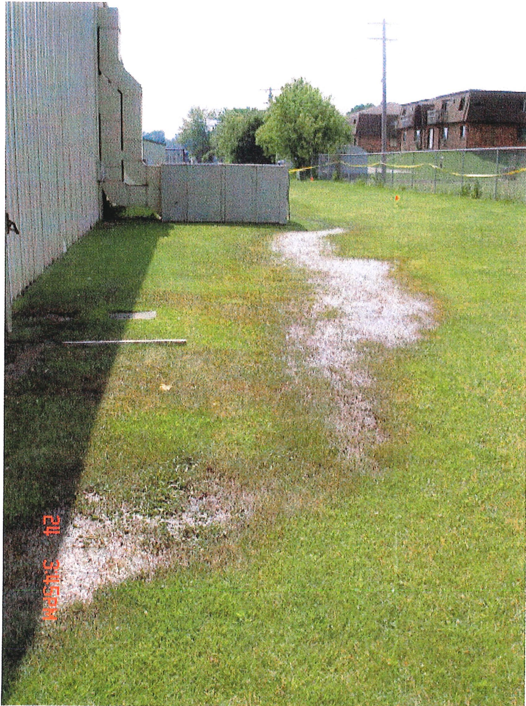
Looking west on north side of building
