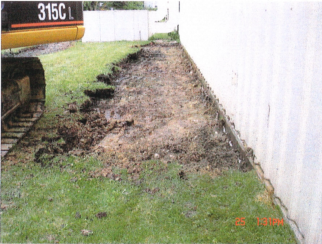
Second excavation on north side adjacent to building
