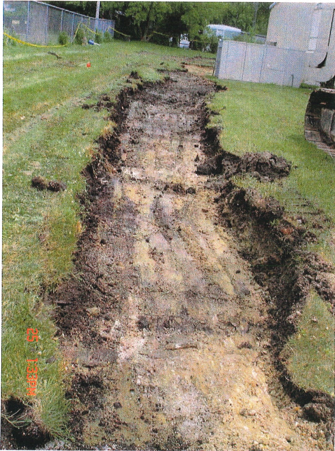
Looking east at excavation on north side of building
