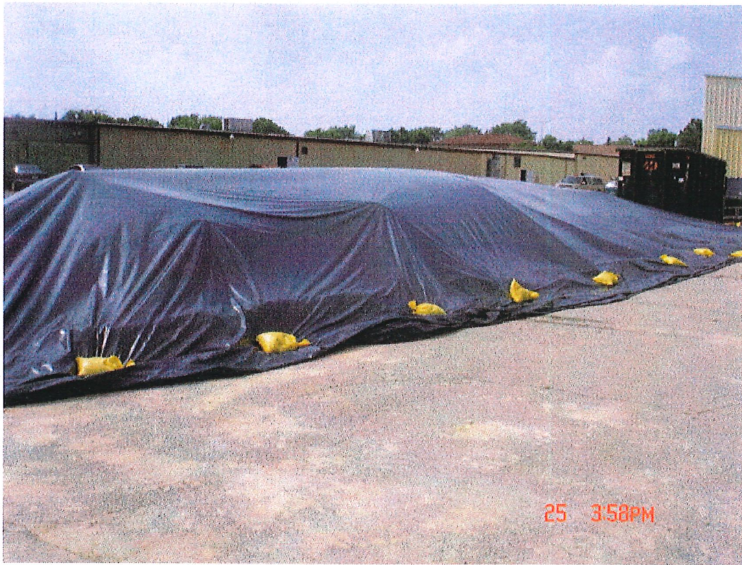
Excavated soil was stockpiled on liner, bermed and covered
