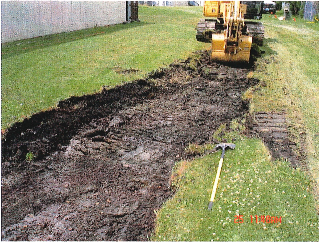
End of first excavation on north side
