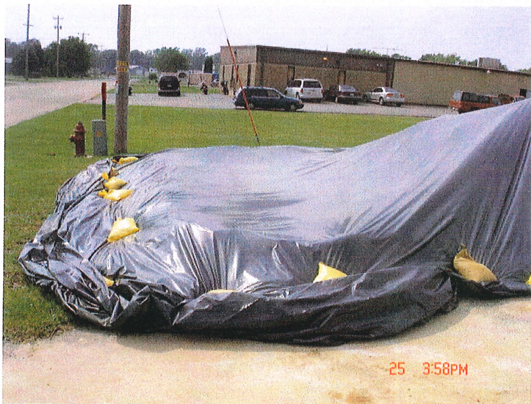
Excavated soil was stockpiled on liner, bermed and covered
