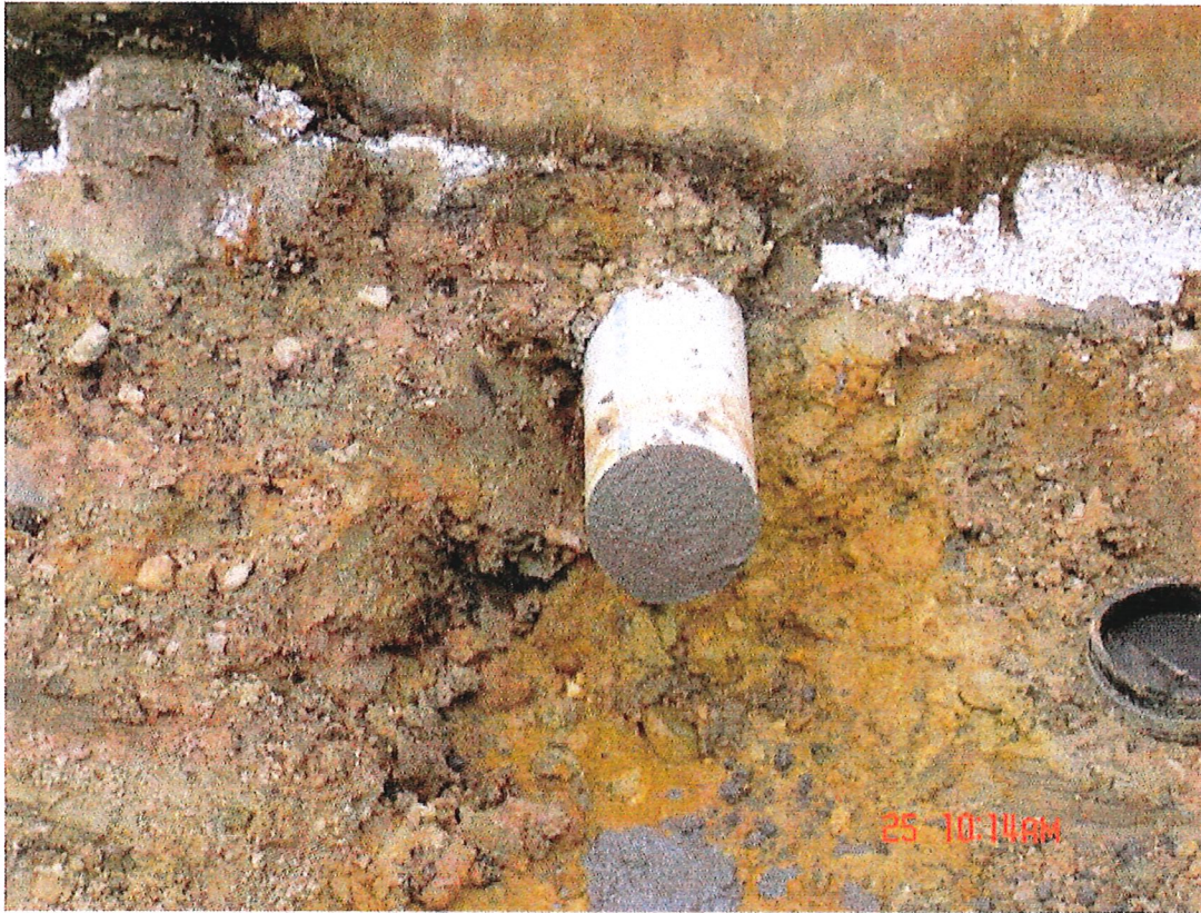
Old floor drain pipe was plugged and capped
