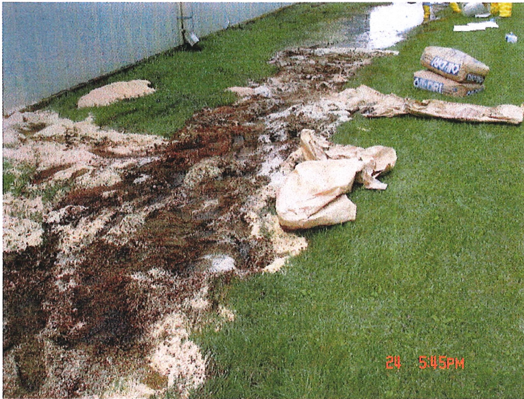
Absorbents were used to contain and recover much of the spilled liquid
