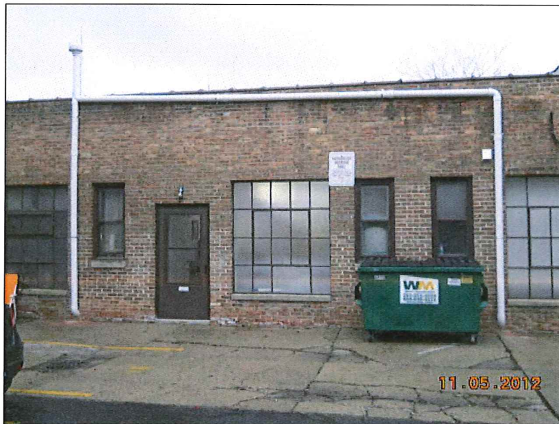
Back of Building Showing As-Built System
