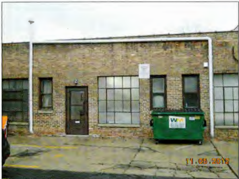
Back of Building Showing As-Built System
