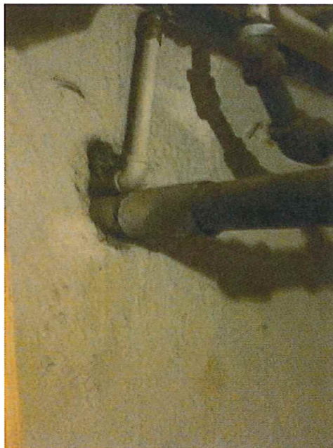
Water line wall penetrations
