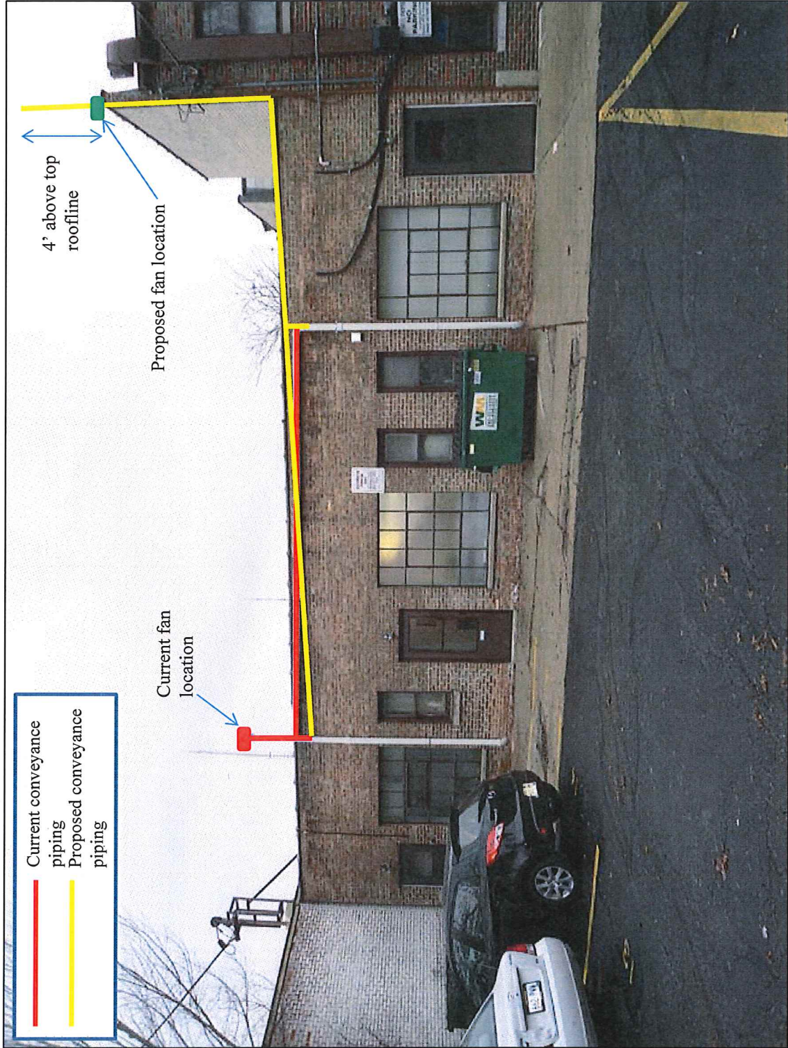
Figure 1 Modification of SSDS Exhaust Stack
