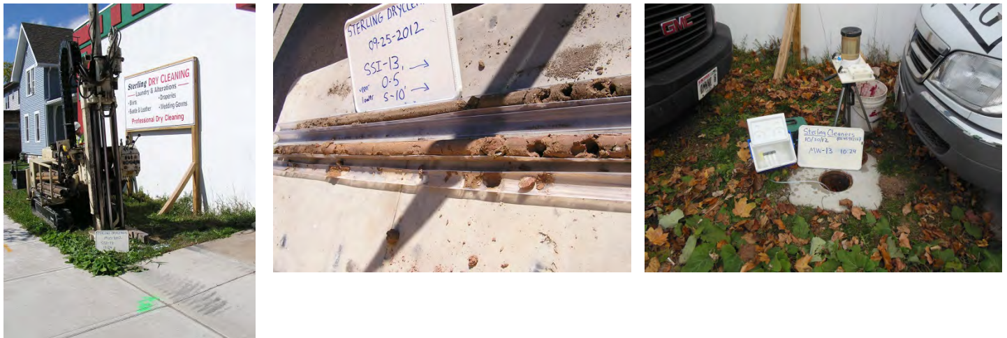
SSI-13 – located on the south side of the SDC facility near the front door. Installed MW-13.
