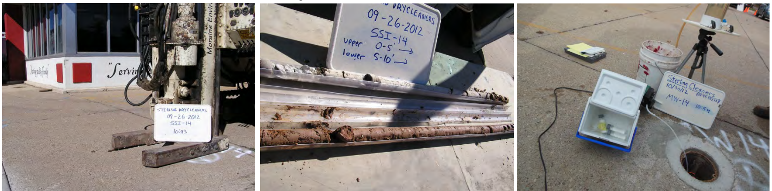
SSI-14 – located southeast of SDC facility. Installed MW-14.
