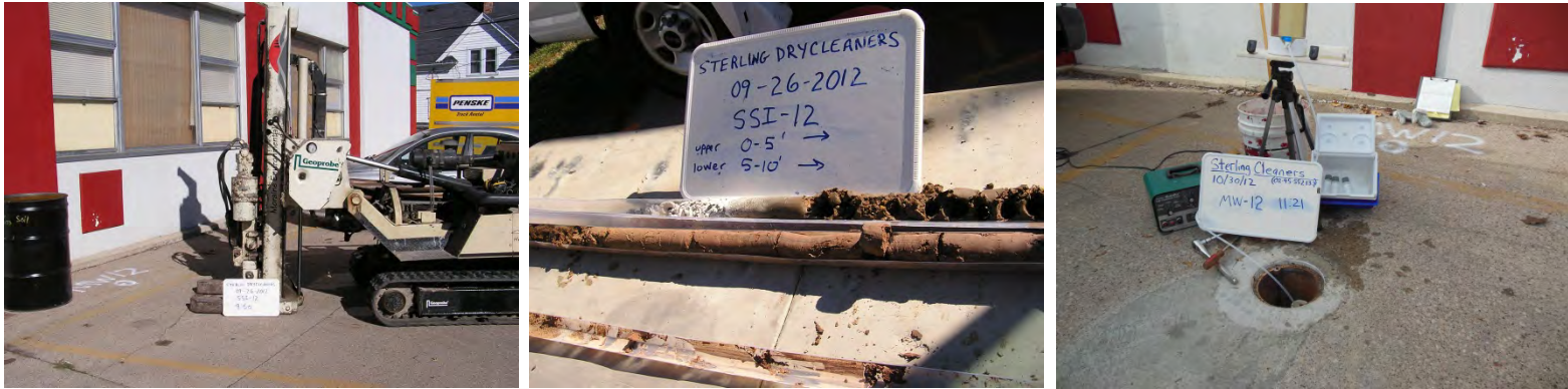
SSI-12 – located on east side of SDC facility. Installed MW-12.
