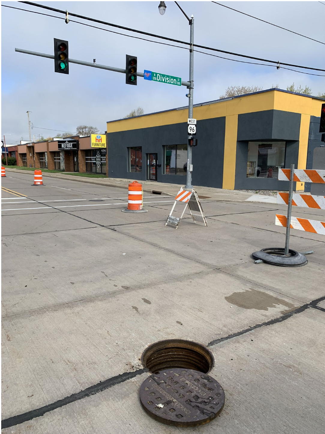
Photo 6: Photo looking northwest at manhole “SAN MH 36-59” with traffic control equipment shown in the background.
