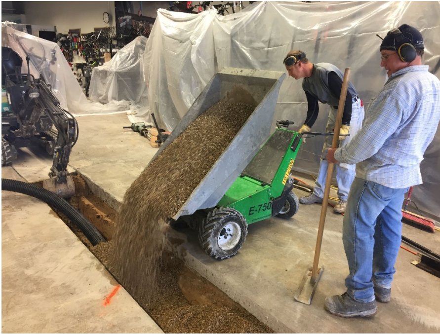
Photo 6: Looking south. Backfilling trench (3/15/20).
