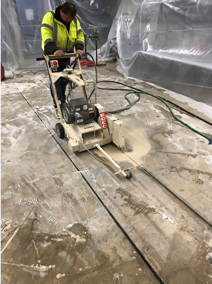
Photo 4: Looking south. Cutting concrete floor (3/14/20).
