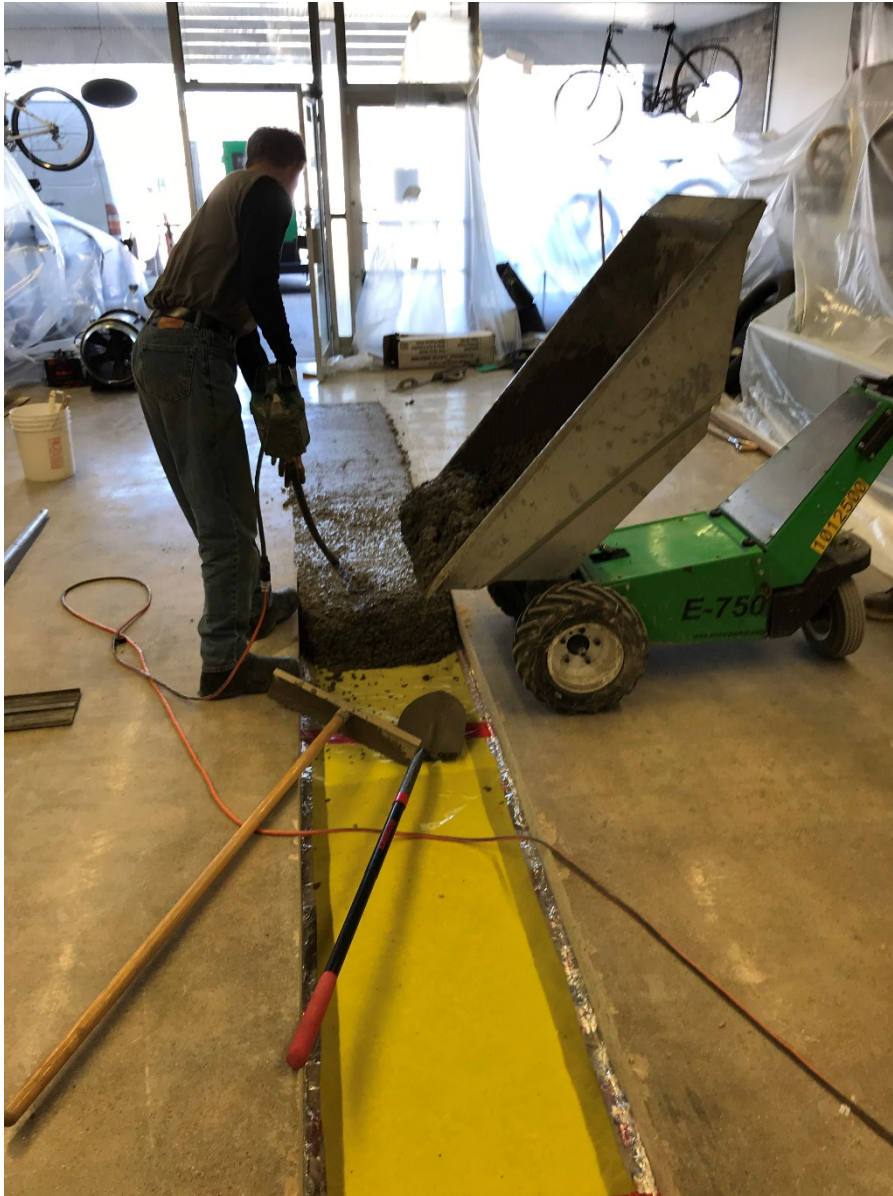
Photo 12: Looking north at vapor barrier and concrete pouring (3/17/20).
