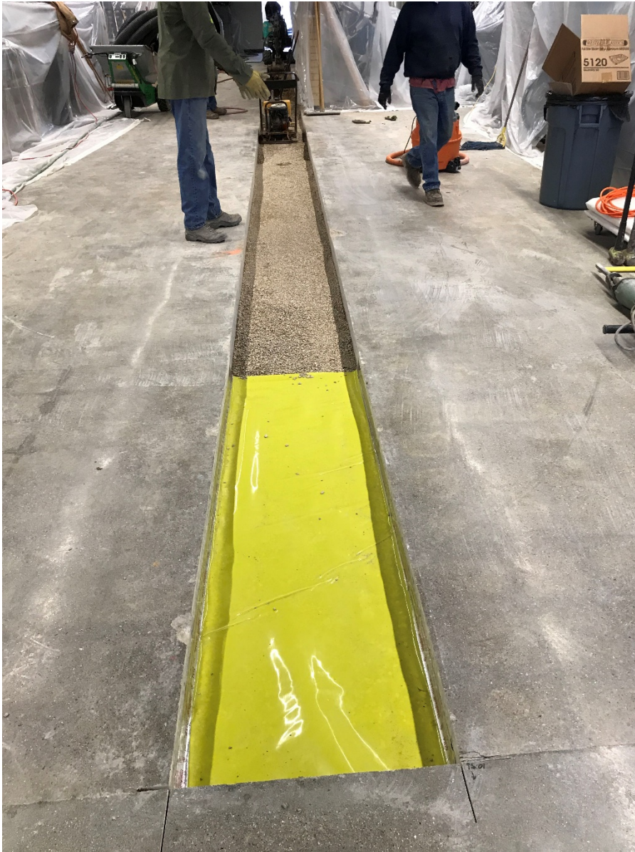
Photo 7: Looking south. Placing Stego Wrap (3/16/20).
