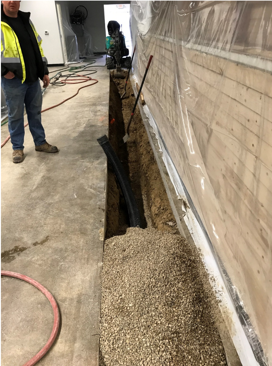
Photo 8: Looking south. Installing perforated piping (3/16/20).
