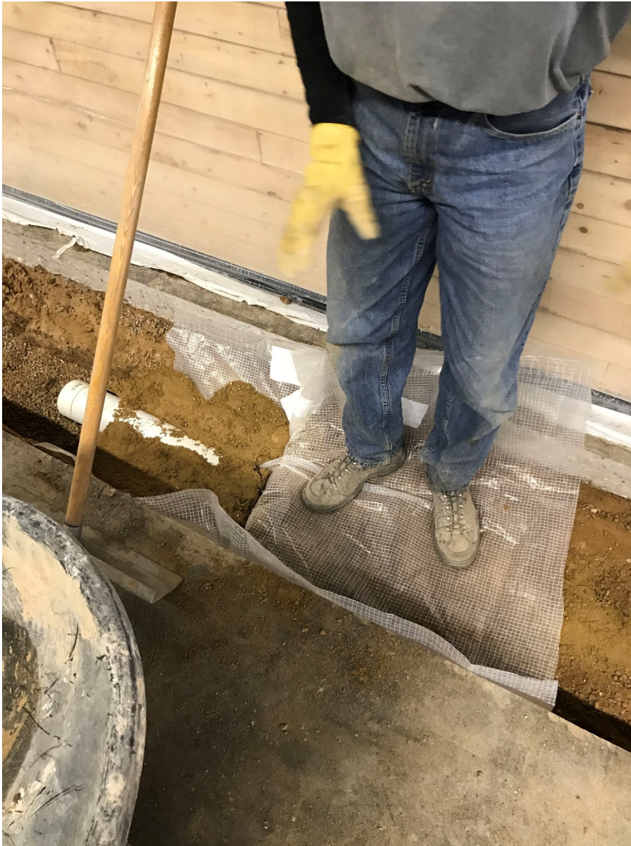
Photo 10: Looking west at seal between north and south perforated pipes (3/16/20).
