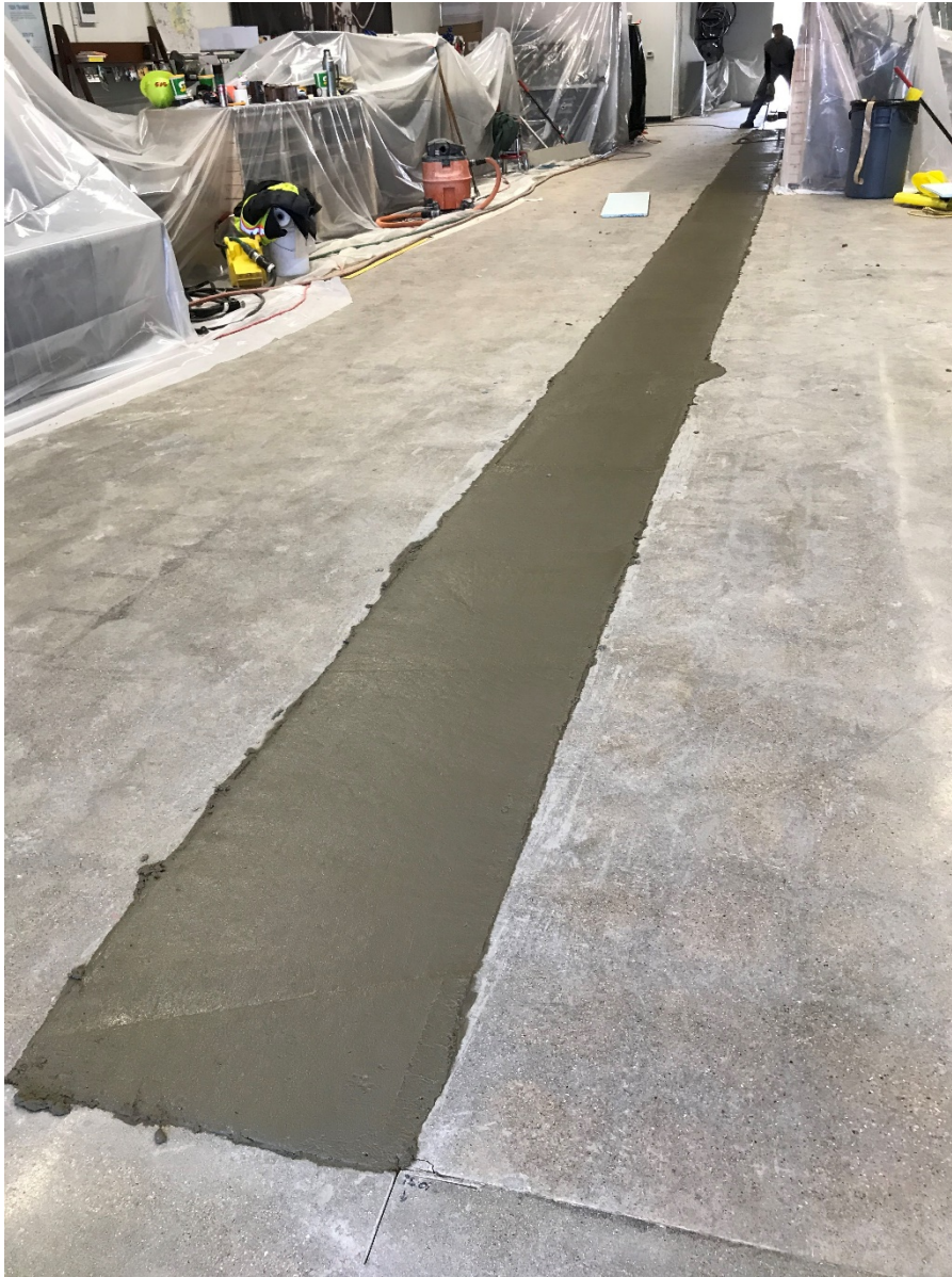
Photo 13: Looking south from front of store at new concrete (3/17/20).
