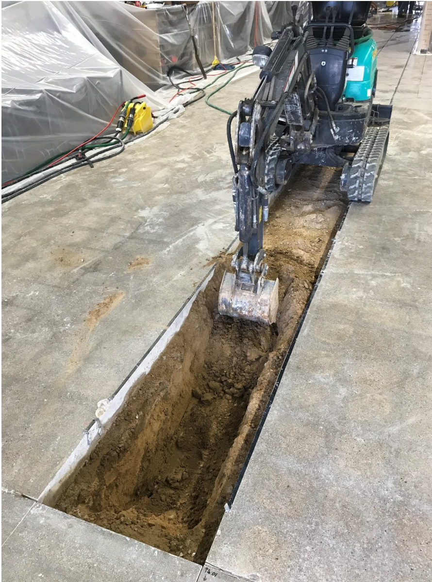
Photo 5: Looking south. Excavating trench (3/15/20).
