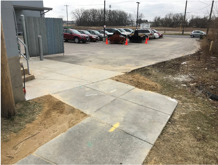
Photo 15: Looking south at roll off bins for trench spoils (left) and clean fine-grained soils used to build ramp (right) (3/23/20).
