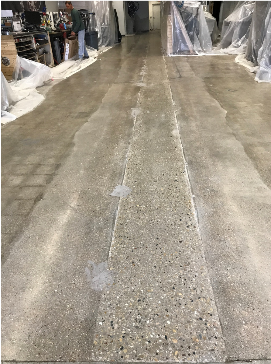
Photo 14: Looking south at concrete after grinding and sealing (3/23/20).
