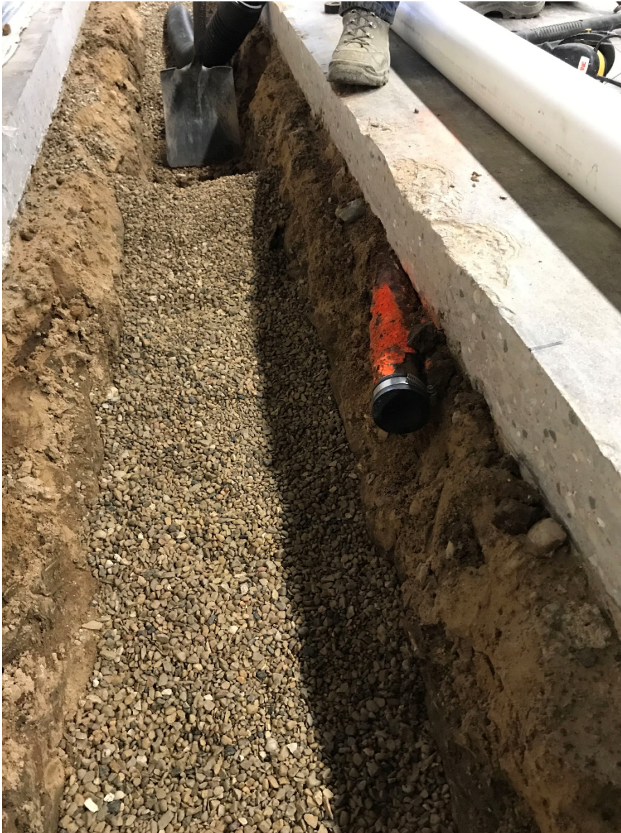
Photo 9: Looking south at abandoned water pipe. Sealed and capped (3/16/20).
