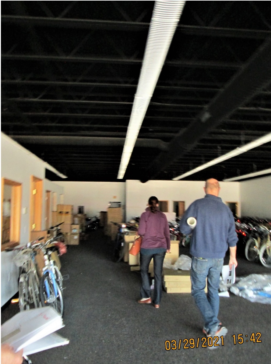
Photo 1: 1117 Vacant – (view to the south/back of unit) used for storage by Dream Bikes. Steel I-beams and trusses exposed in ceiling are the same as thorough out the building.
