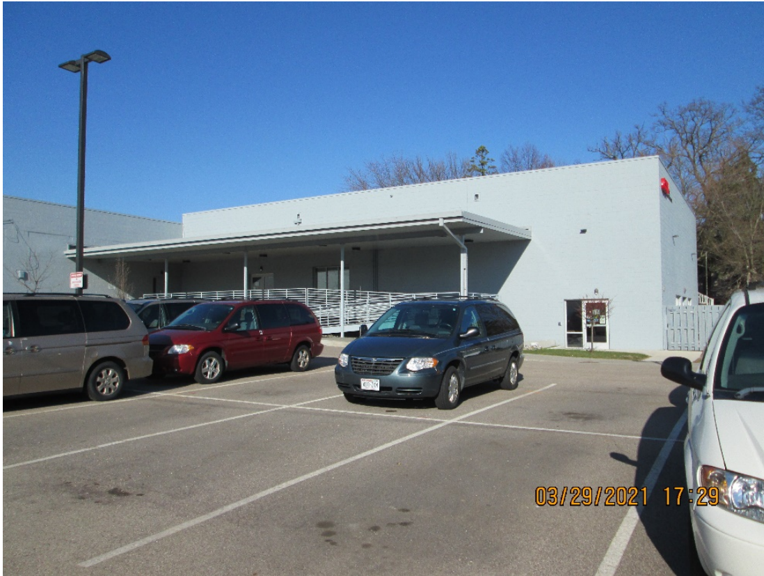
Photo 10: CSN 1151 Vapor mitigation system Fan #8 to be mounted on exterior wall above south end of canopy.
