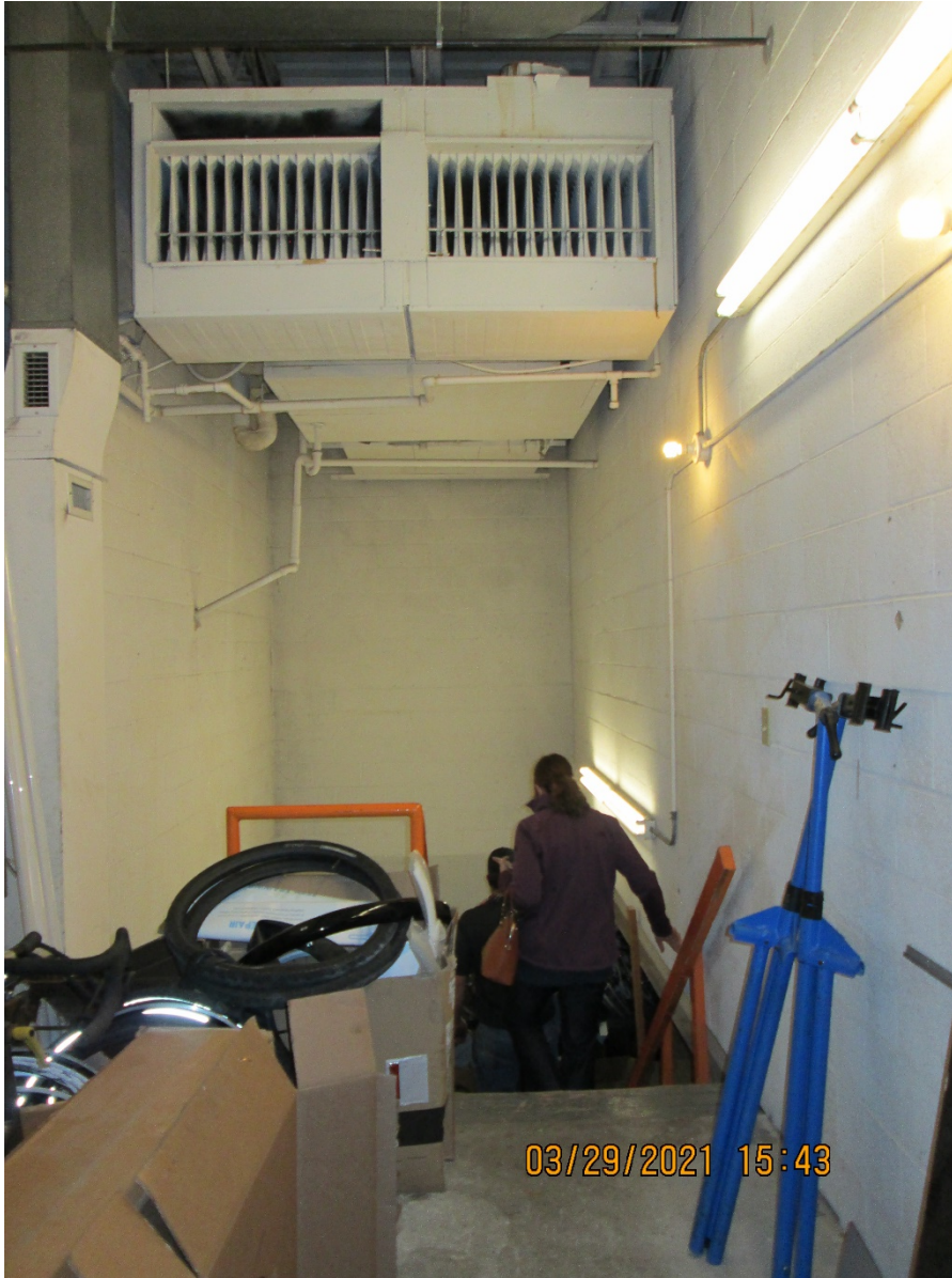
Photo 2: Stair well at back of Unit 1117. Access to pick-up points 1-4.
