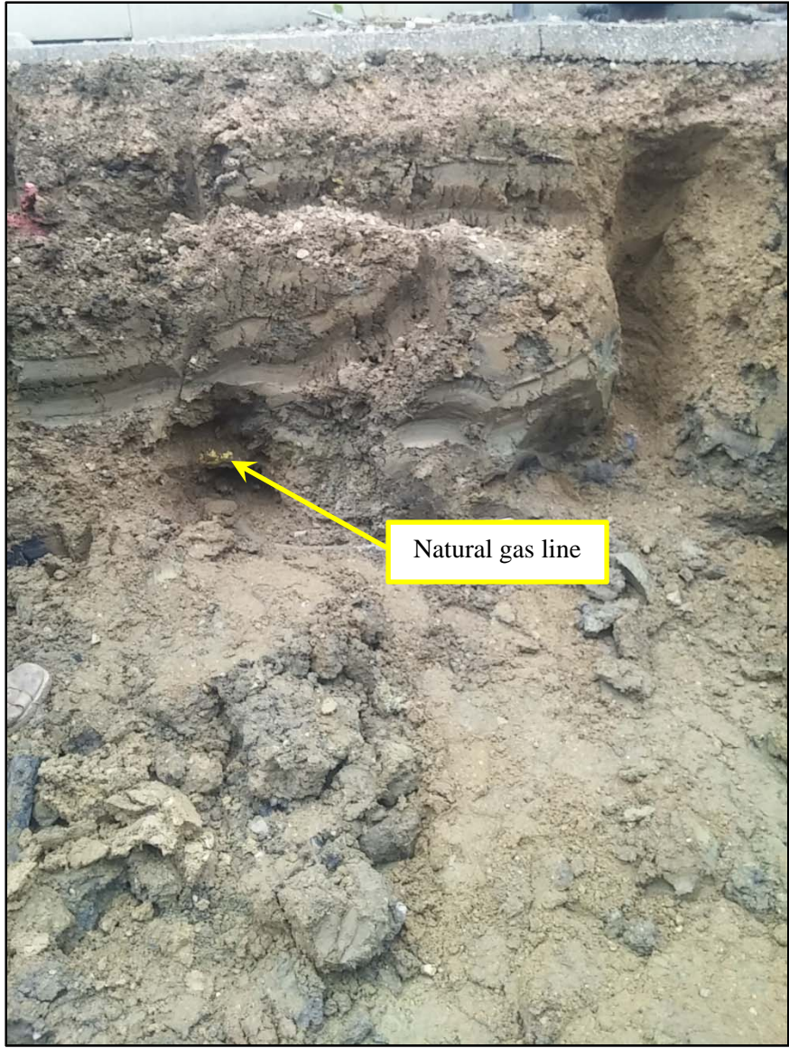
North wall of exterior excavation area 1
