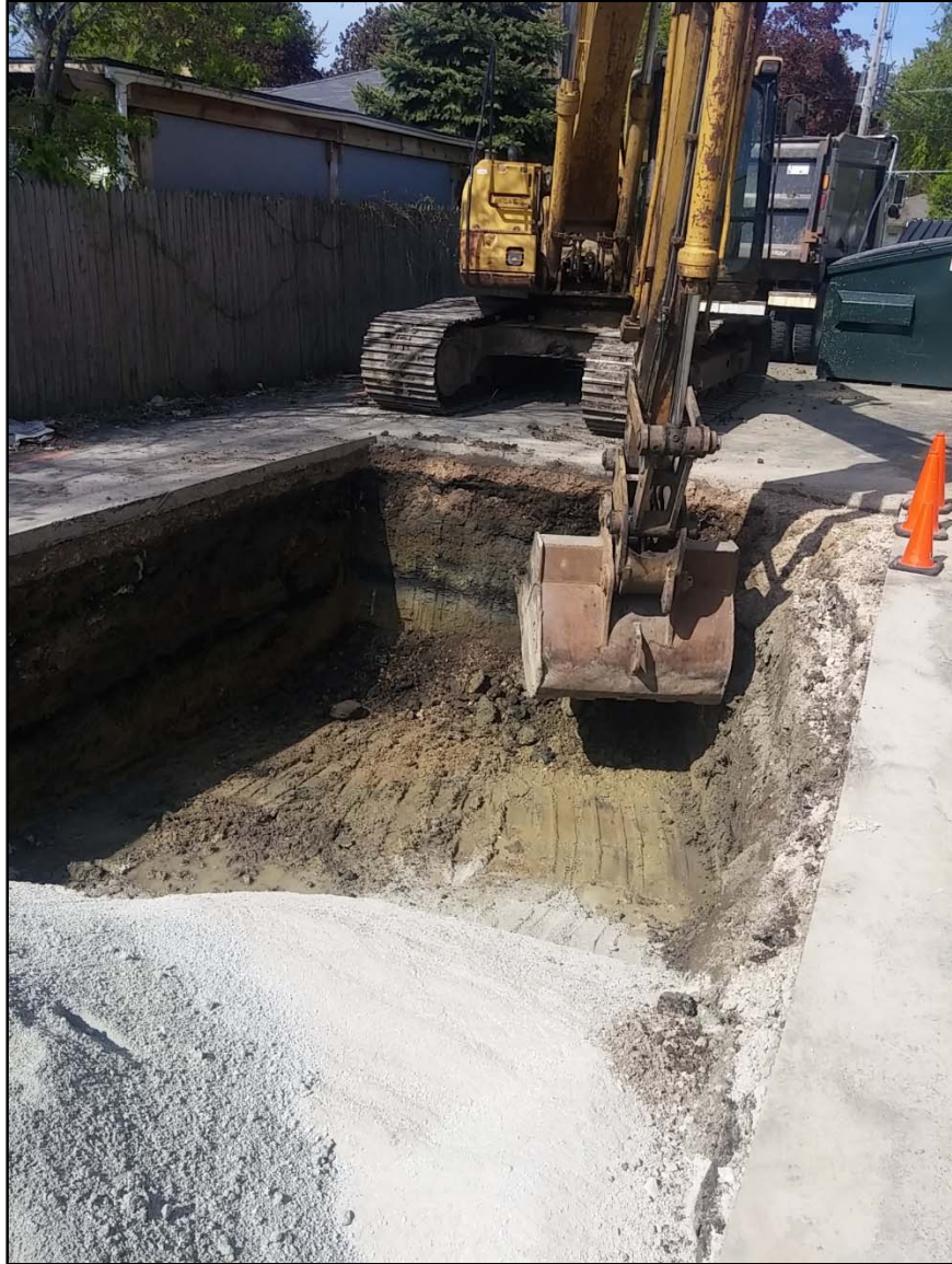
West wall of exterior excavation area 1
