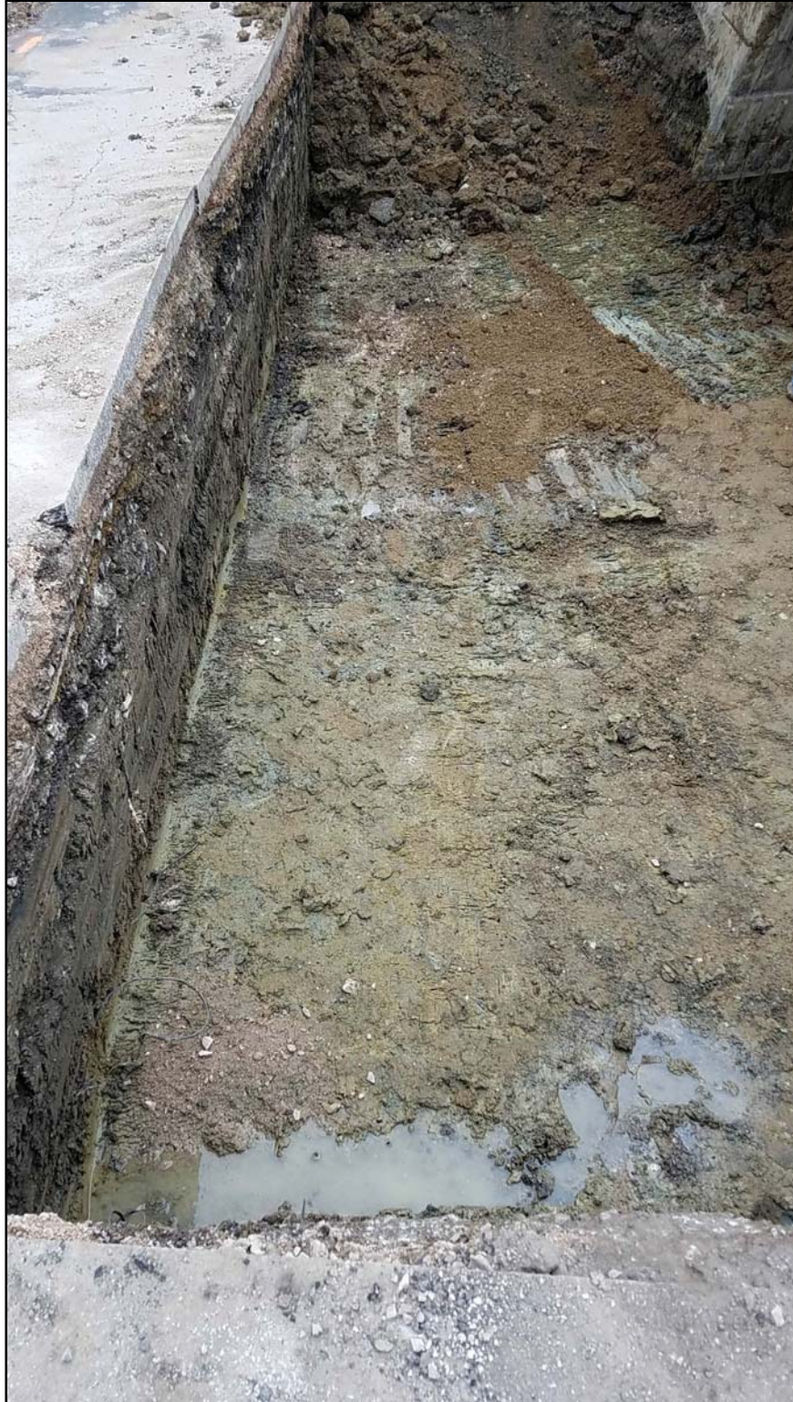
Floor of exterior excavation area 1
