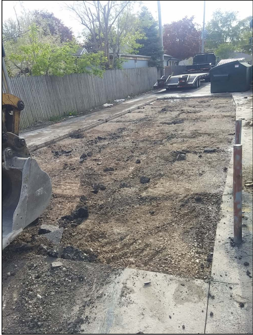
Exterior excavation area 1 asphalt removal
