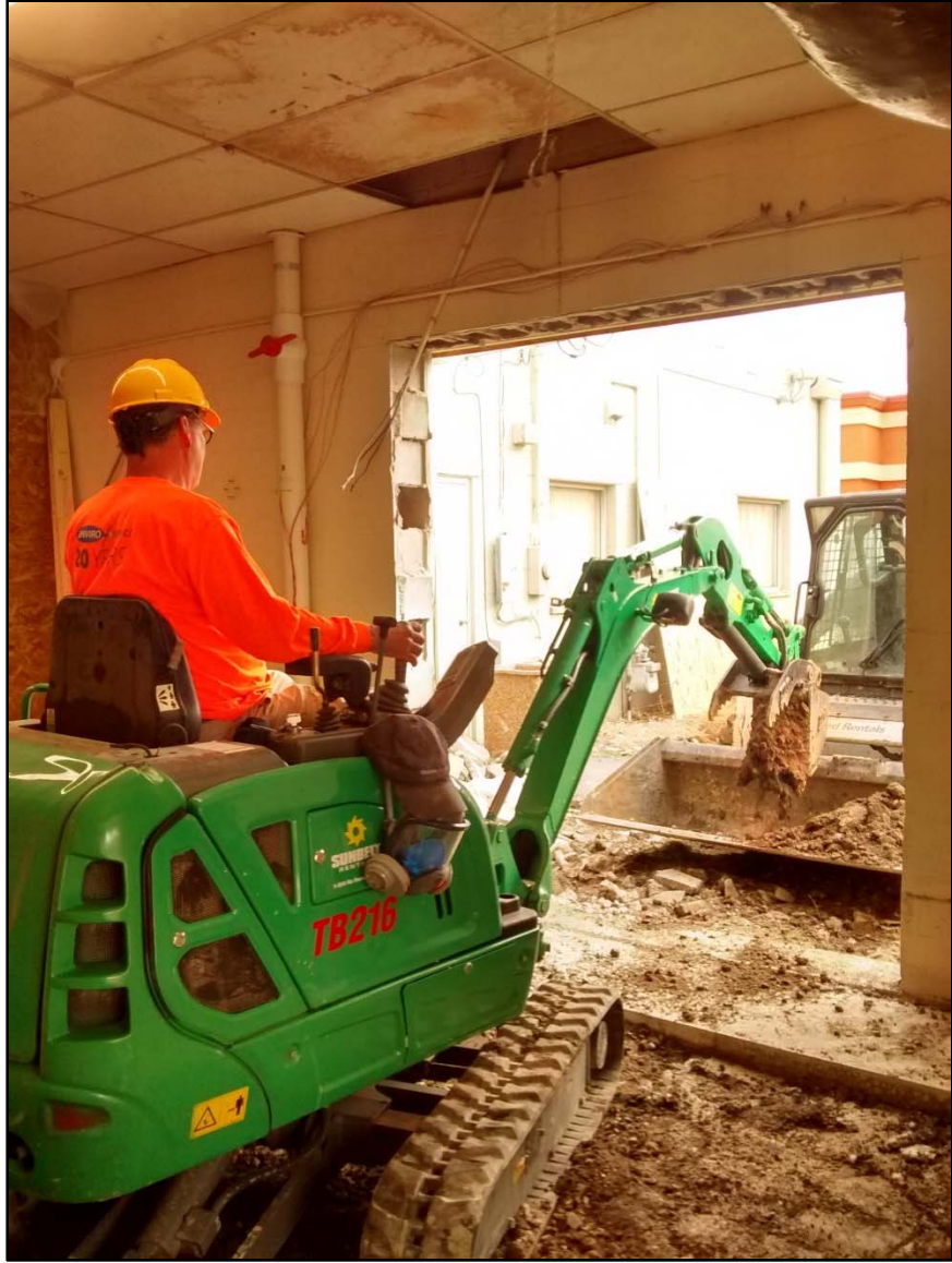
Interior excavation access
