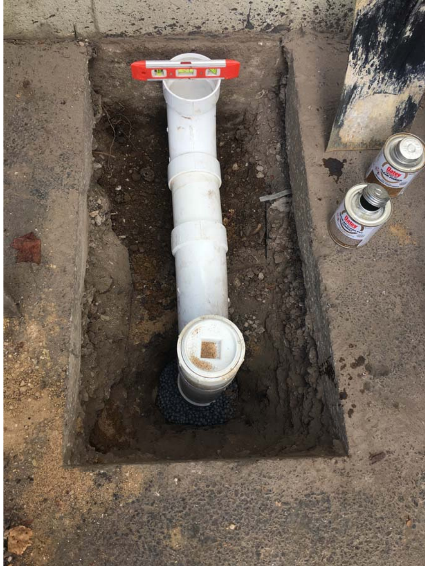
Typical soil vapor extraction wellhead design.
