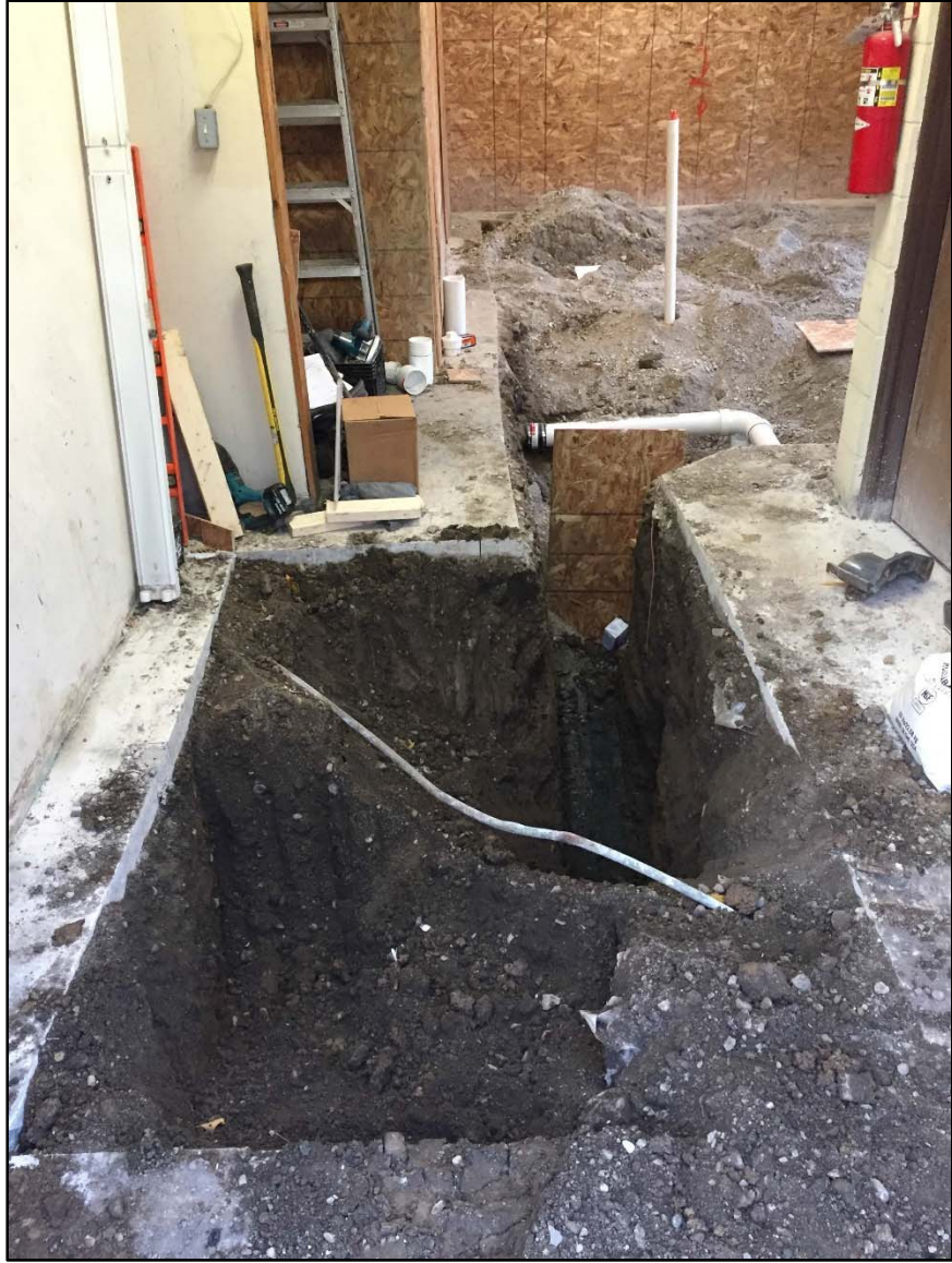
Southern part of interior excavation
