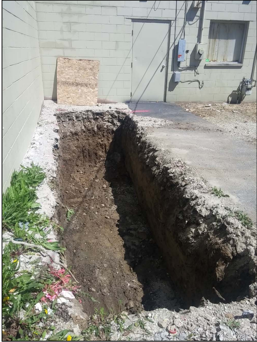
Exterior excavation area 2
