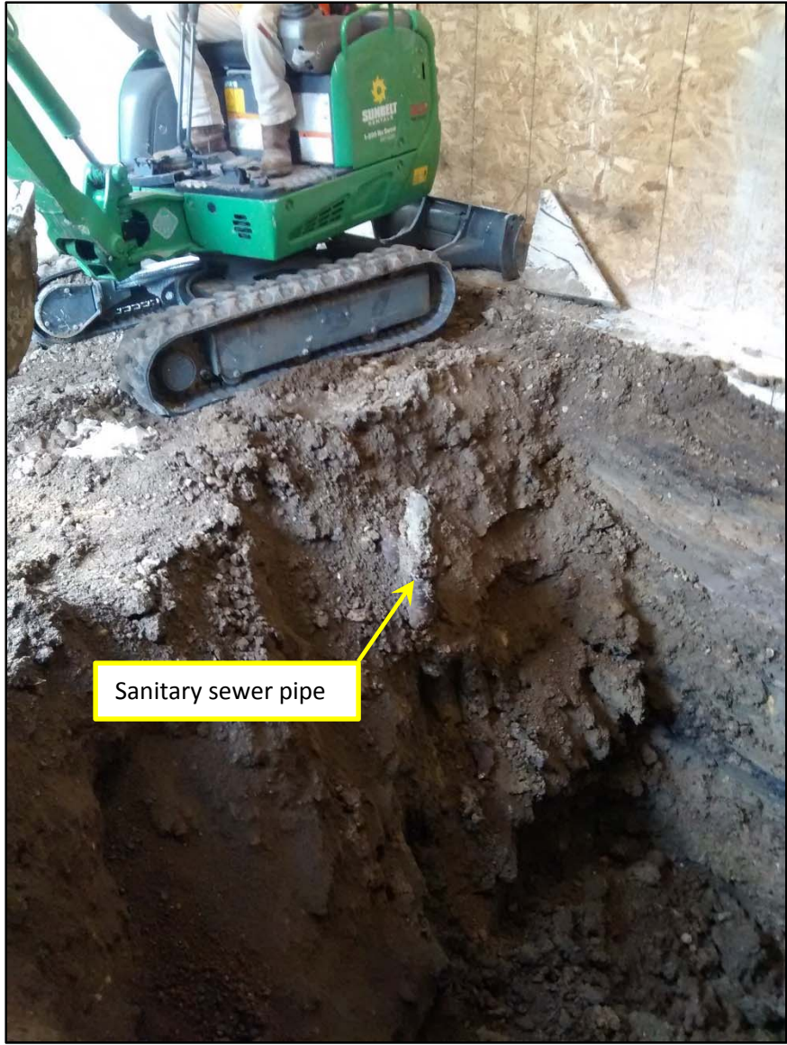
Interior excavation and cast iron sewer pipe
