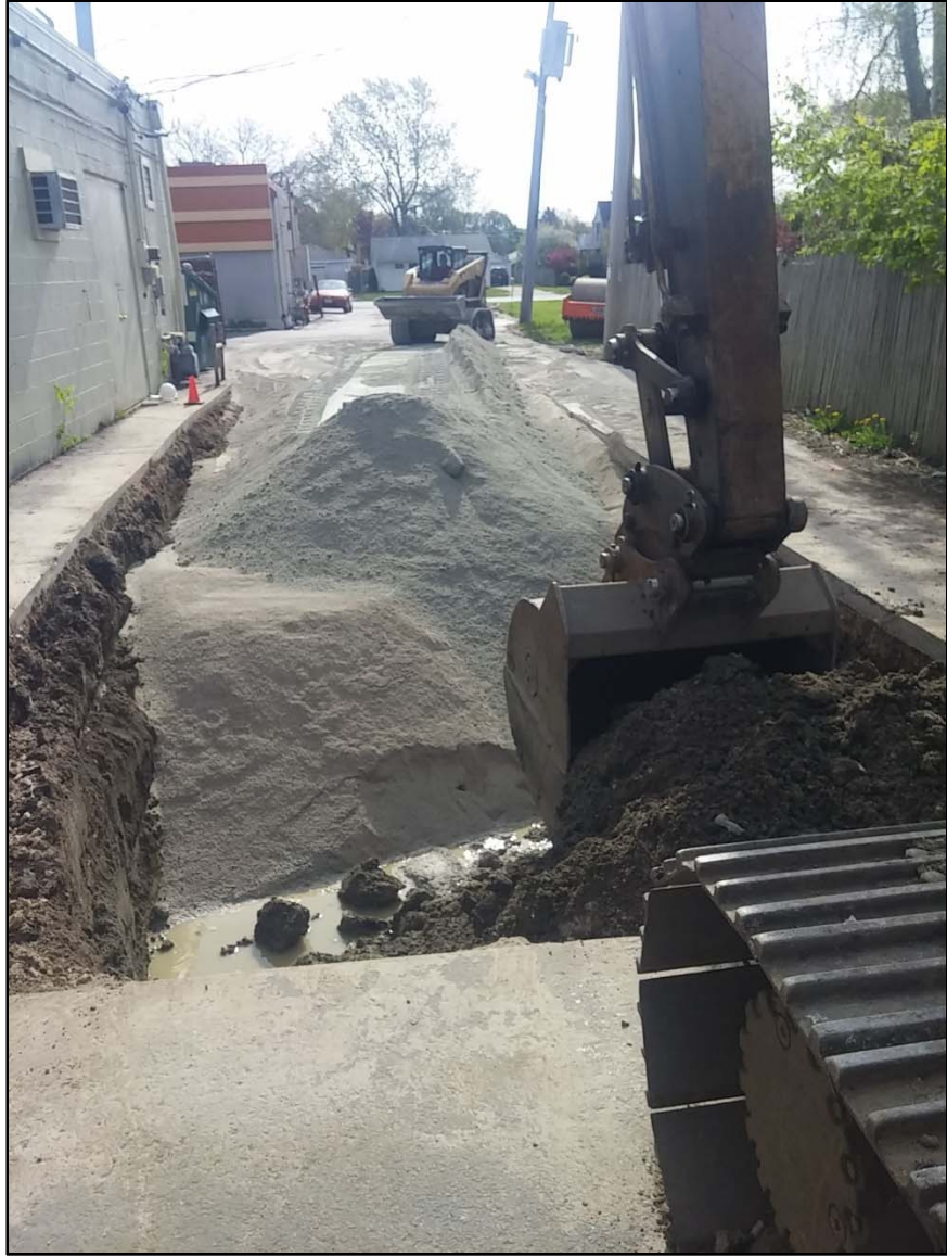
Exterior excavation area 1 backfill
