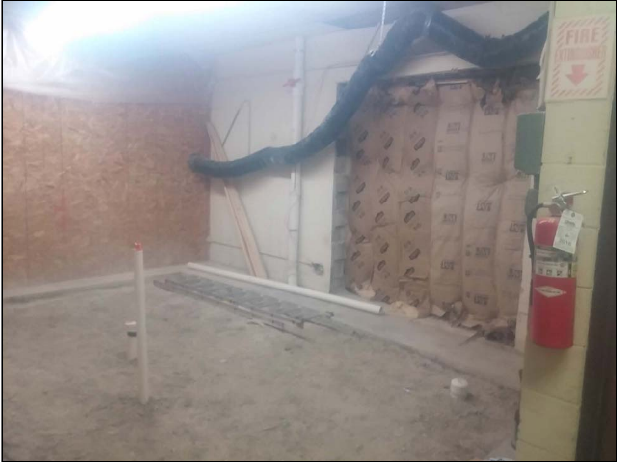
Interior excavation backfill and compaction completed
