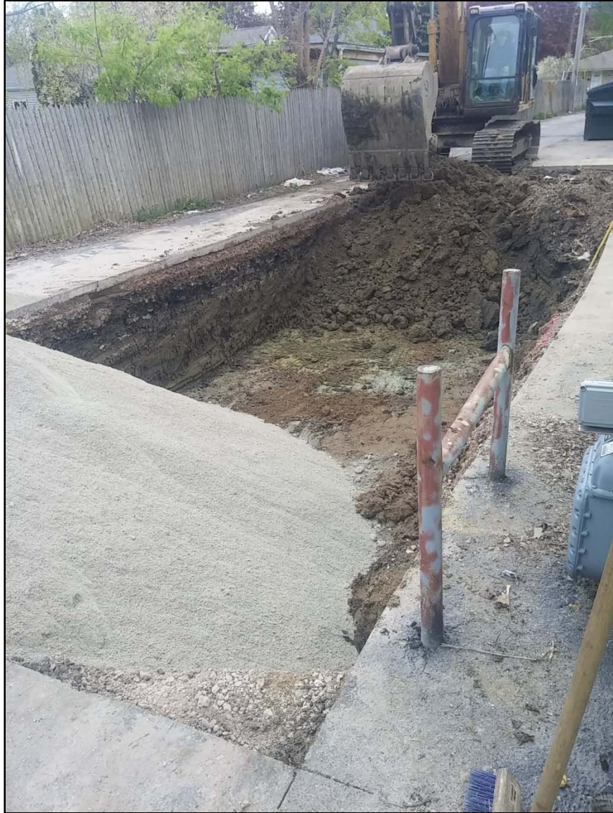
Overview of exterior excavation area 1
