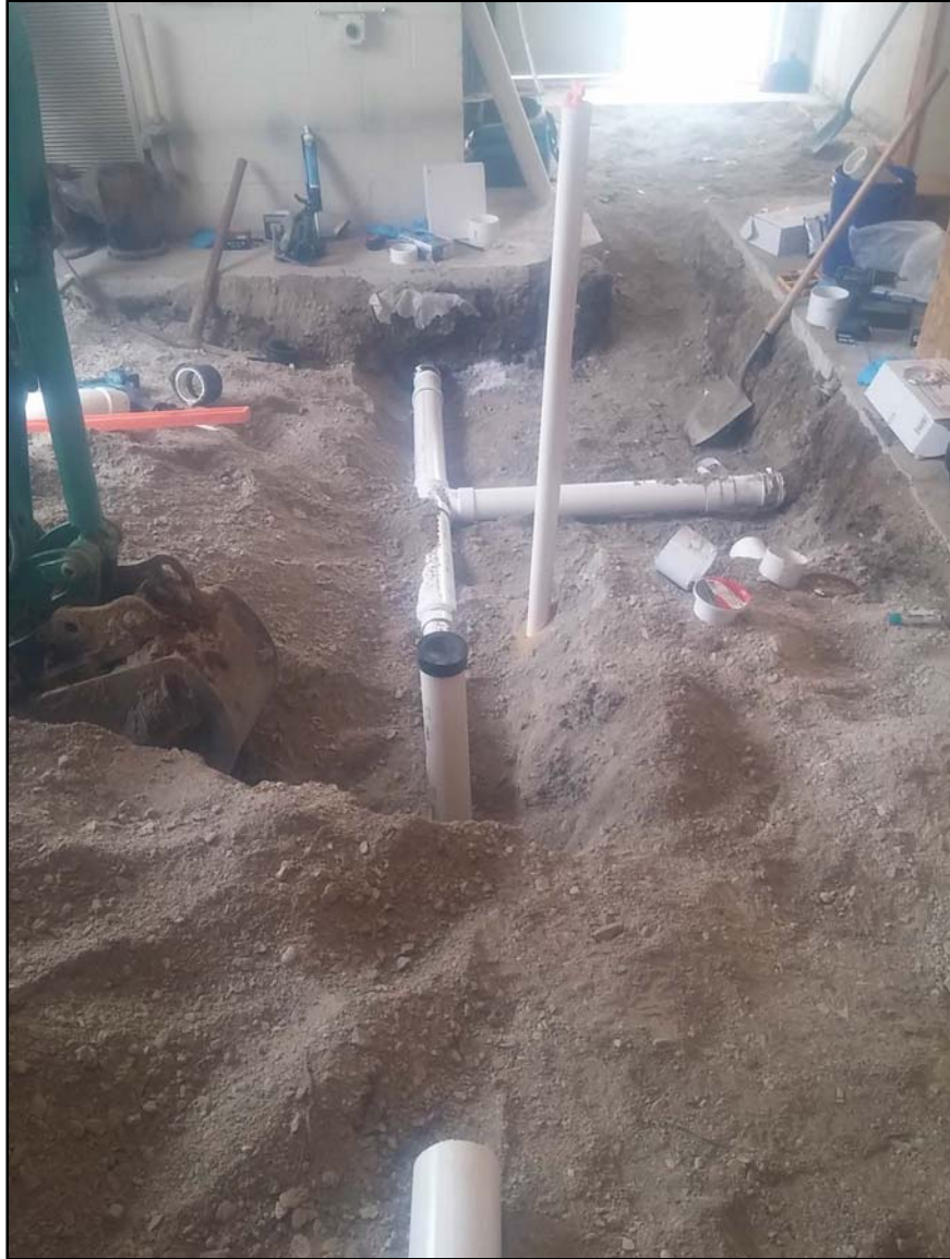
Replacement sewer laterals and contingency injection point
