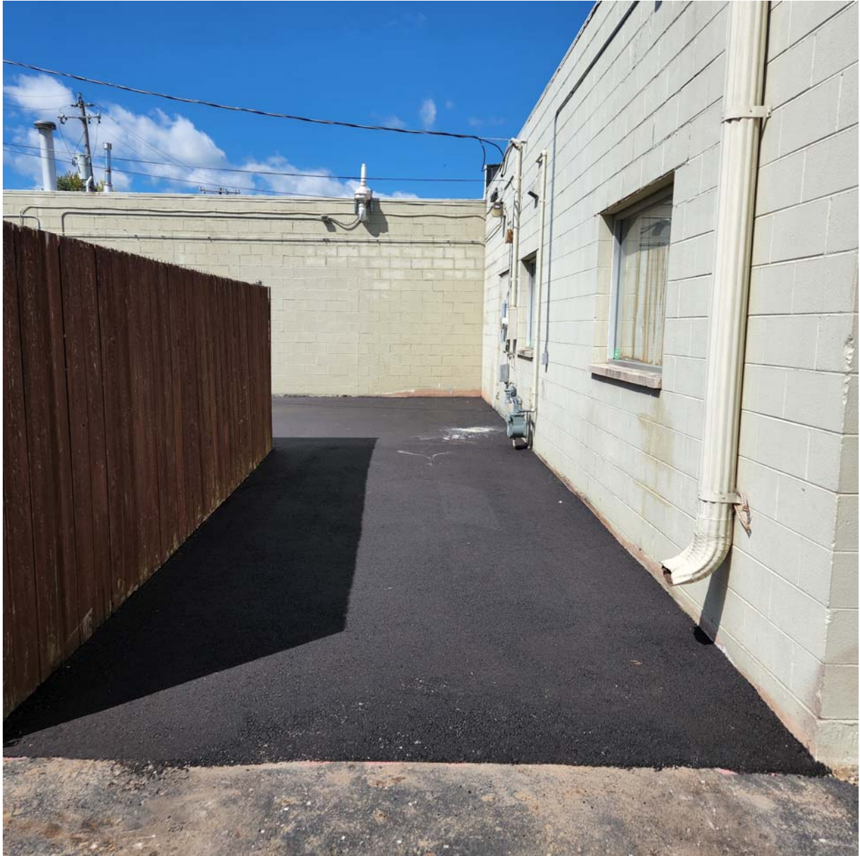
Asphalt cap south of 3909 52 nd Street, facing west.
