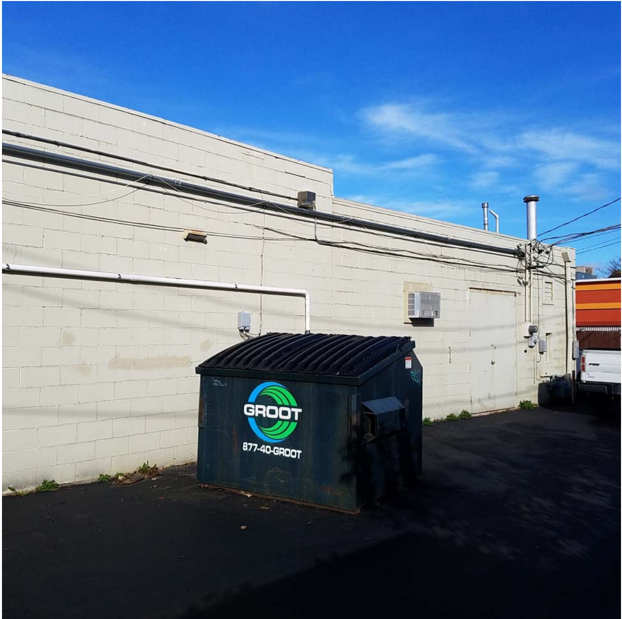
South side of the 3917 52 nd Street building, facing northeast
