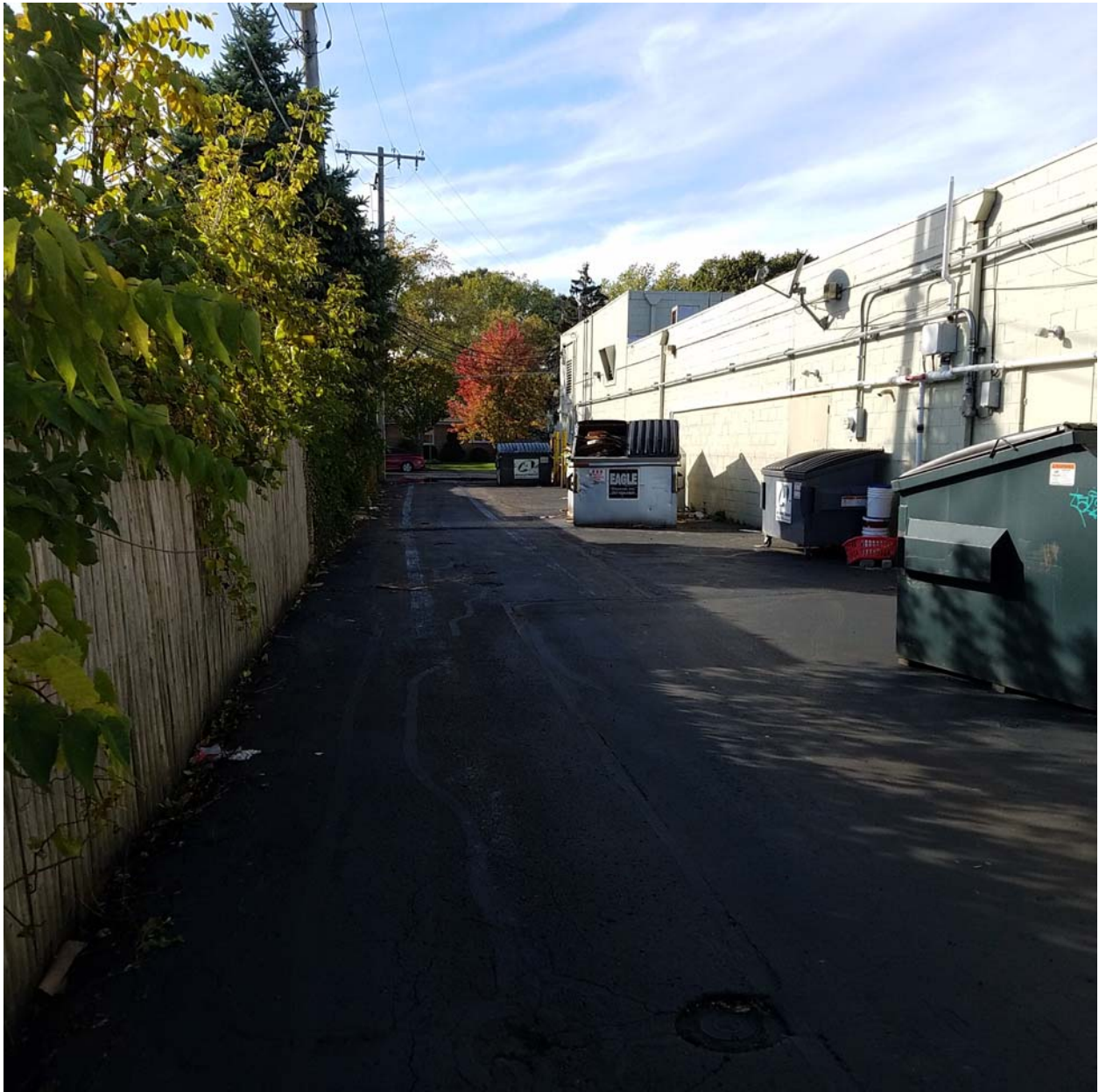
Overview of alleyway portion of the asphalt cap south of 3917 52 nd Street, facing west
