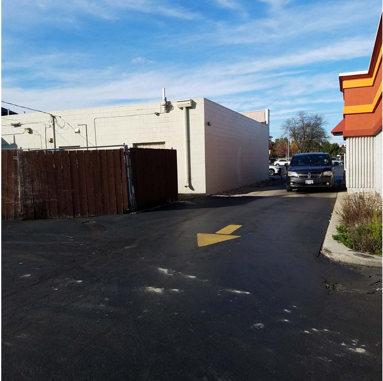
Asphalt cap between the 3909 and 3907 52 nd Street buildings, facing north
