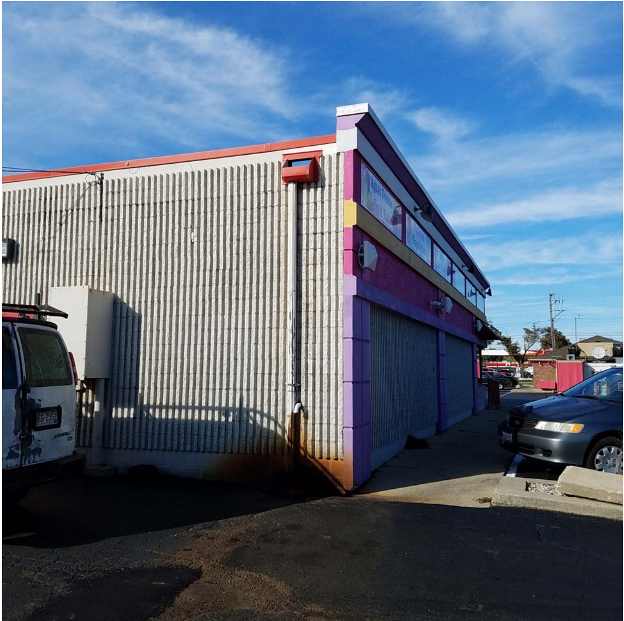
East side of the 3907 52 nd Street building, facing north
