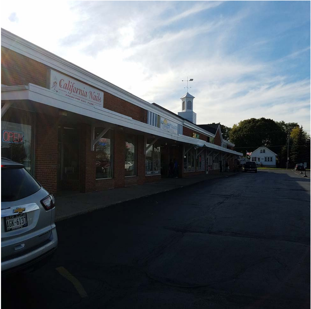
North side of the 3909 and 3917 52 nd Street commercial buildings, facing west
