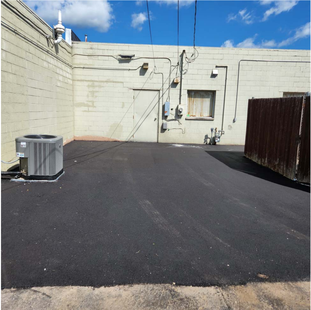
Asphalt cap east of Site building, facing north.
