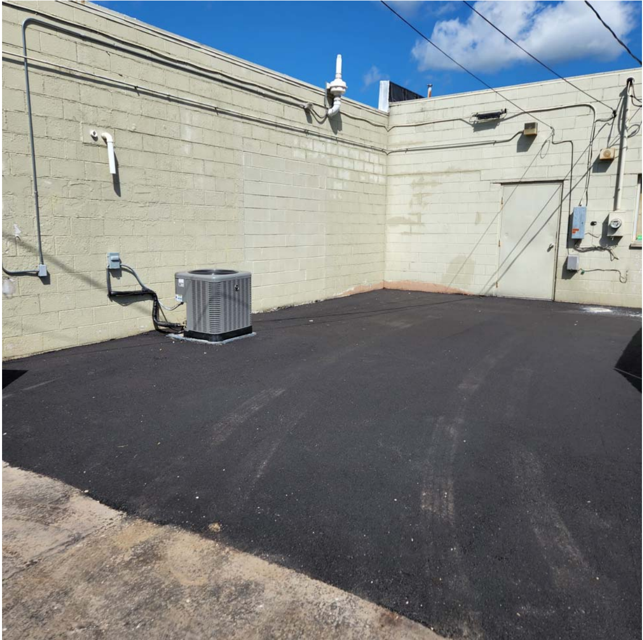
Asphalt cap east of Site building, facing northwest.
