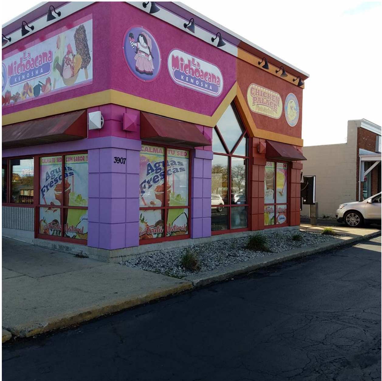
North side of the 3907 52 nd Street building, facing southwest
