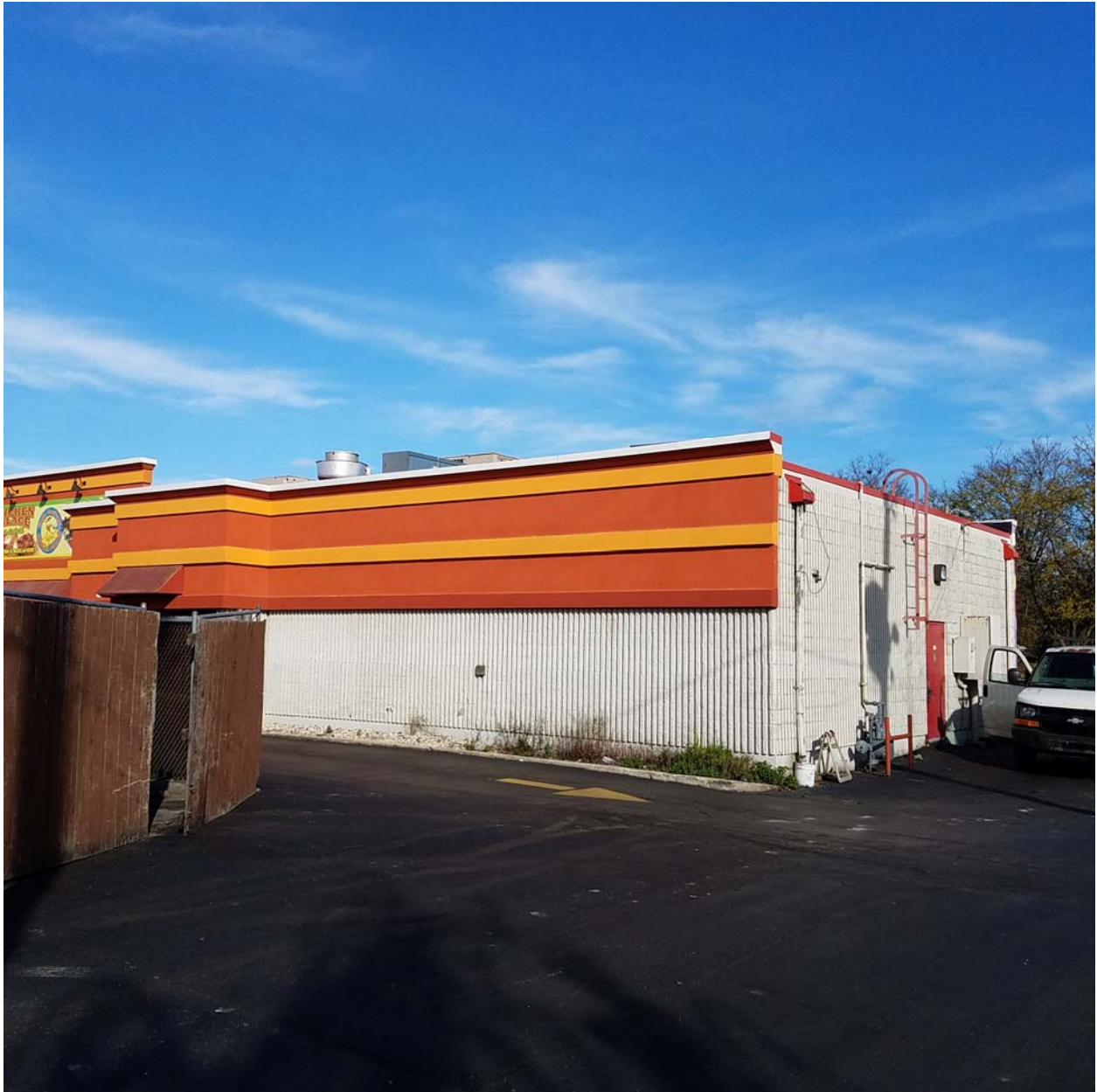
West side of the 3907 52 nd Street building, facing northeast
