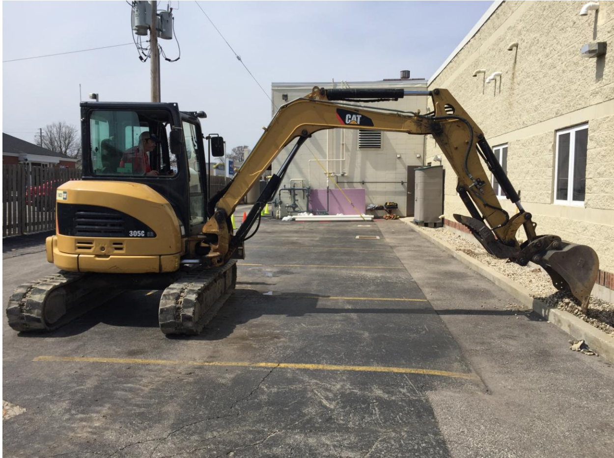
Trench excavation along south wall of building
