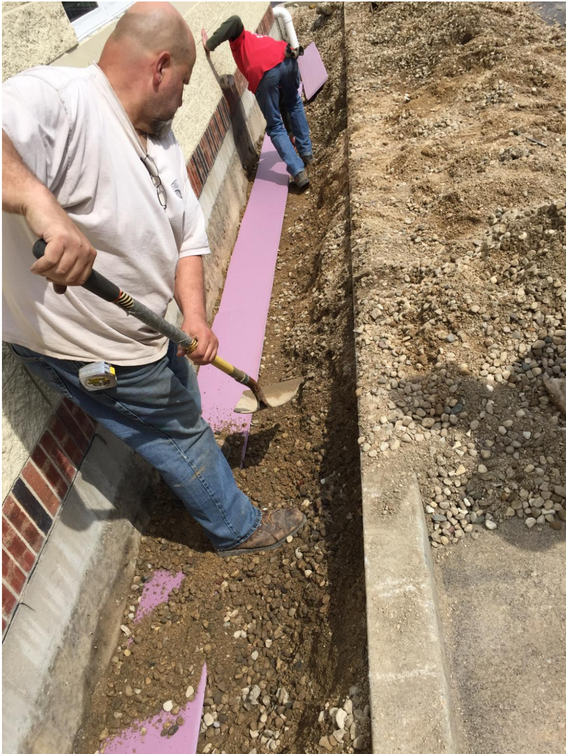
Adding 1 inch purple foam board (Polystyrene) over the conveyance line sections that are 2 feet bgs.
