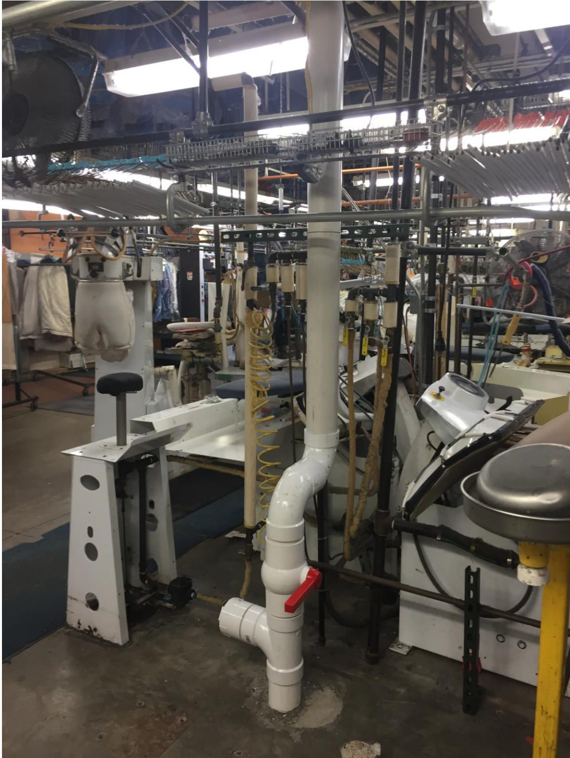
SVE-2 with ball valve and clean out.
