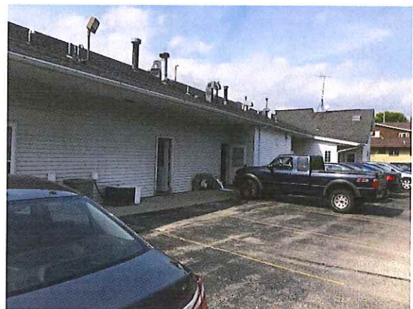
Photo #4 Existing Building and Pavement Cap
