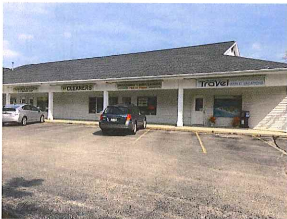
Photo #3 Existing Building and Pavement Cap
