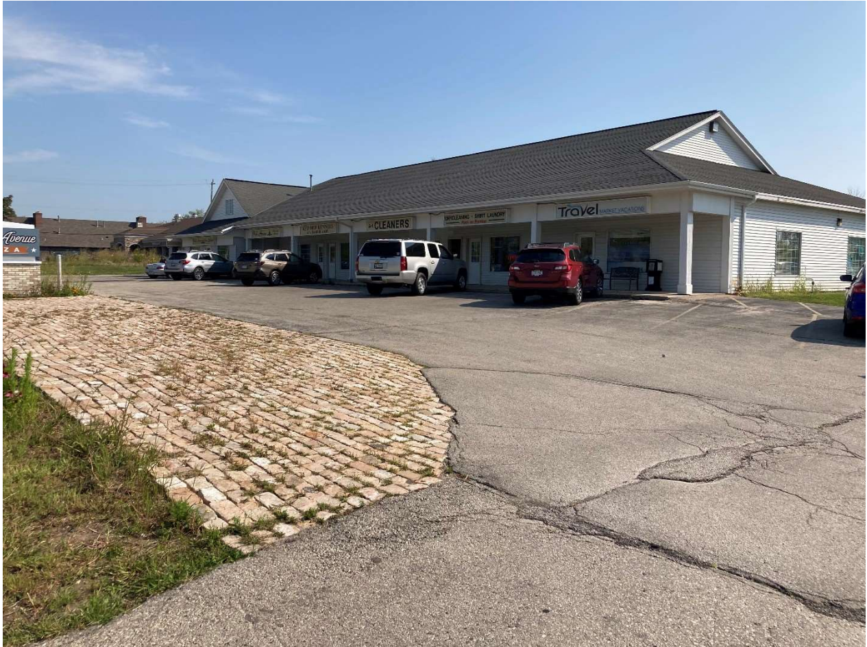
Existing Building and Pavement Cap – Front of Building
