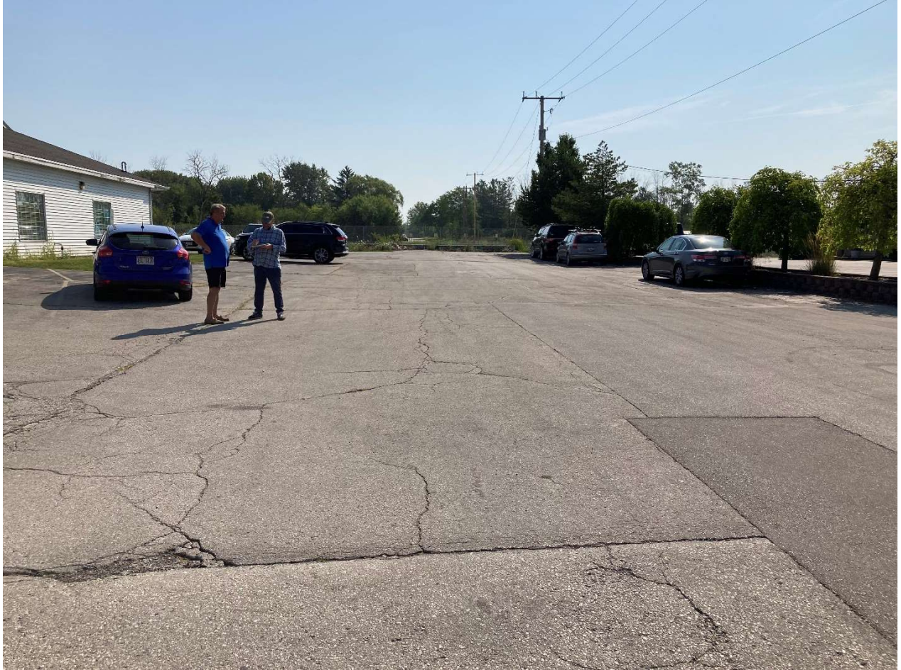
South side of property – Existing building and pavement cap
