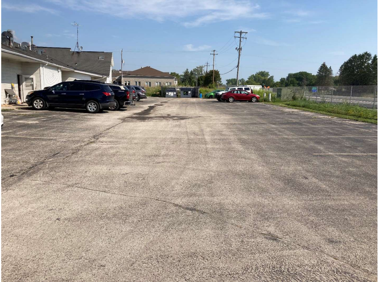
Existing building and pavement cap – East side, Rear of building
