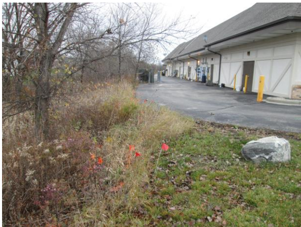
Photo #3 View of west side of strip mall looking north. G-Town Cleaners tenant space on southwest building corner. (Photo Taken: 11/12/2012)
