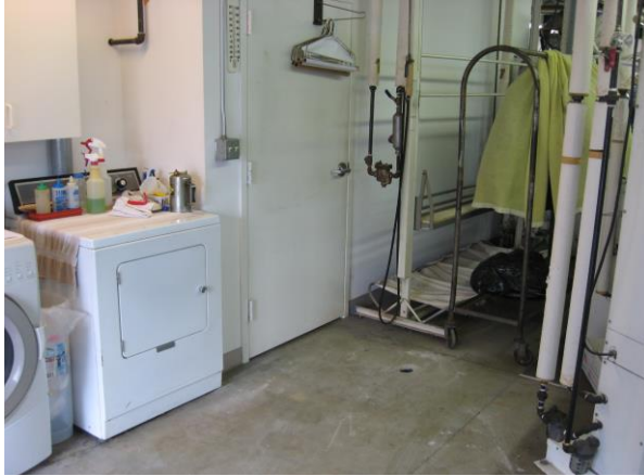
Photo #1 View of building interior and soil boring P-1 location. (Photo taken: 11/6/2008).
