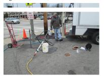
chloroethene (TCE), continued to increase in monitoring well MW-2. As a result Terracon proposed to directly inject a carbon/hydrogen donor amendment and an inoculum containing CVOC-degrading bacteria in an
