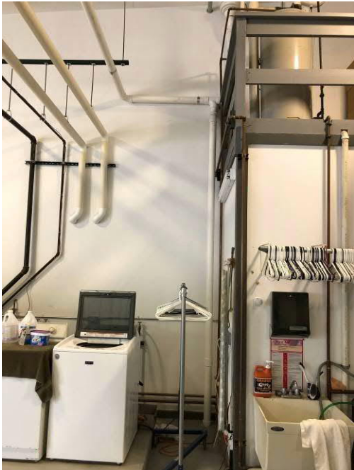
Photo #5 Photograph of northern drop-point component part of the SSDS.
