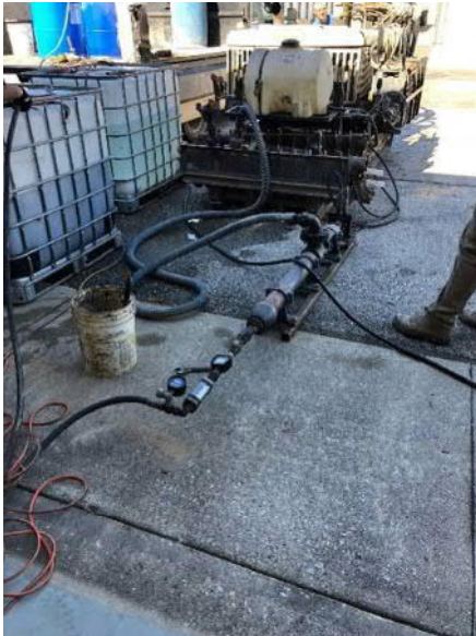
Photo #3 Photograph of injection pumping and mixing set up.
