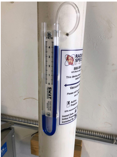
Photo #7 Photograph of the U-Tube manometer vacuum measuring device on the southern drop-point.
