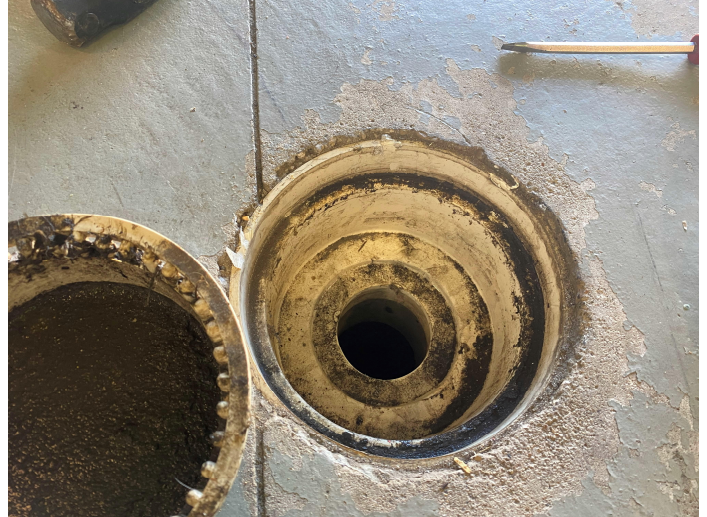
Photo #2 North floor drain.
